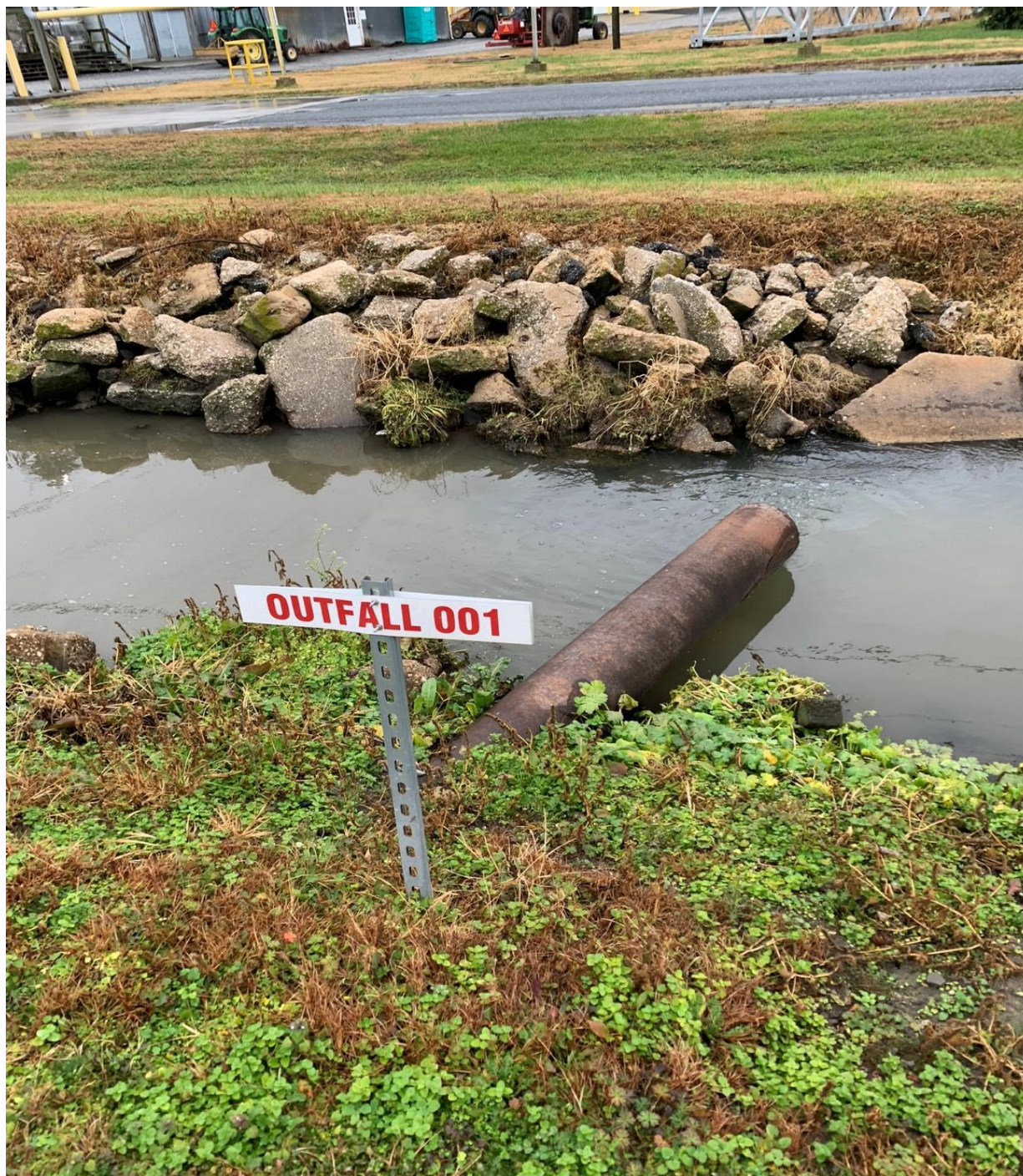
Figure 8. View of the final effluent – Outfall 001
