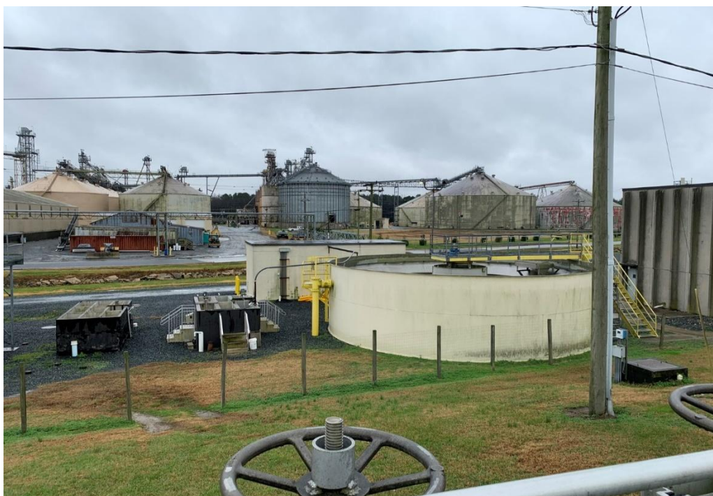
Figure 7. View of one of the clarifier (currently empty for maintenance) and the chlorine contact chamber
