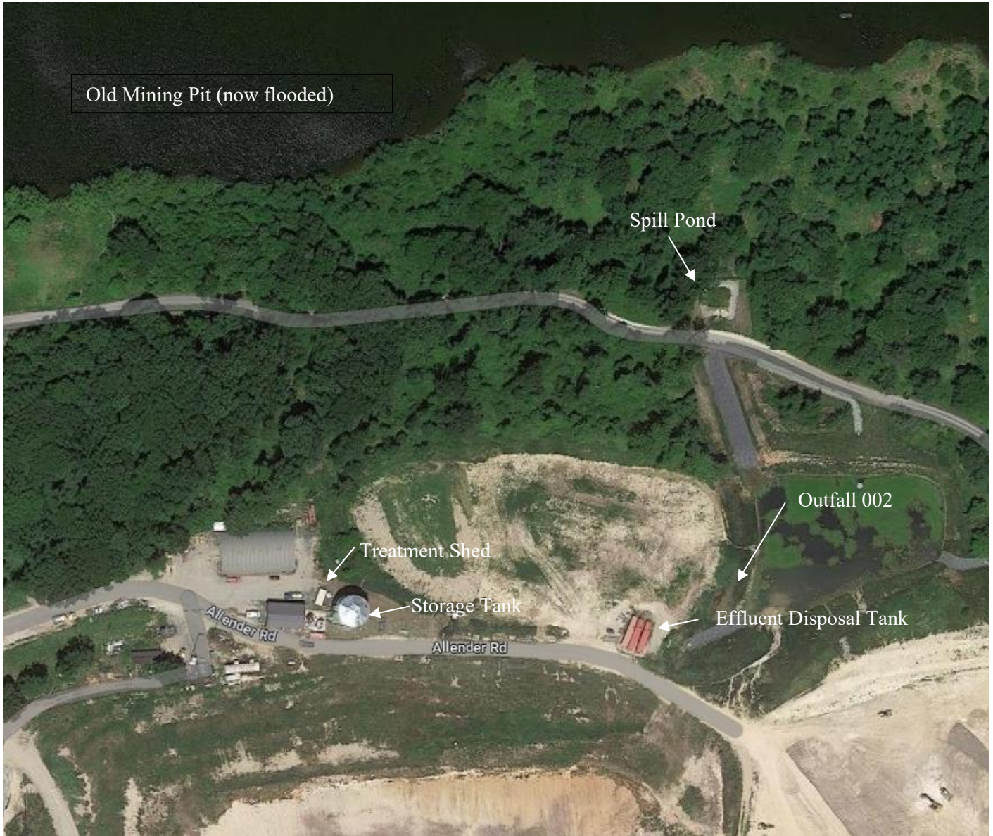
Figure 2. Treatment Facility and Outfall 002
