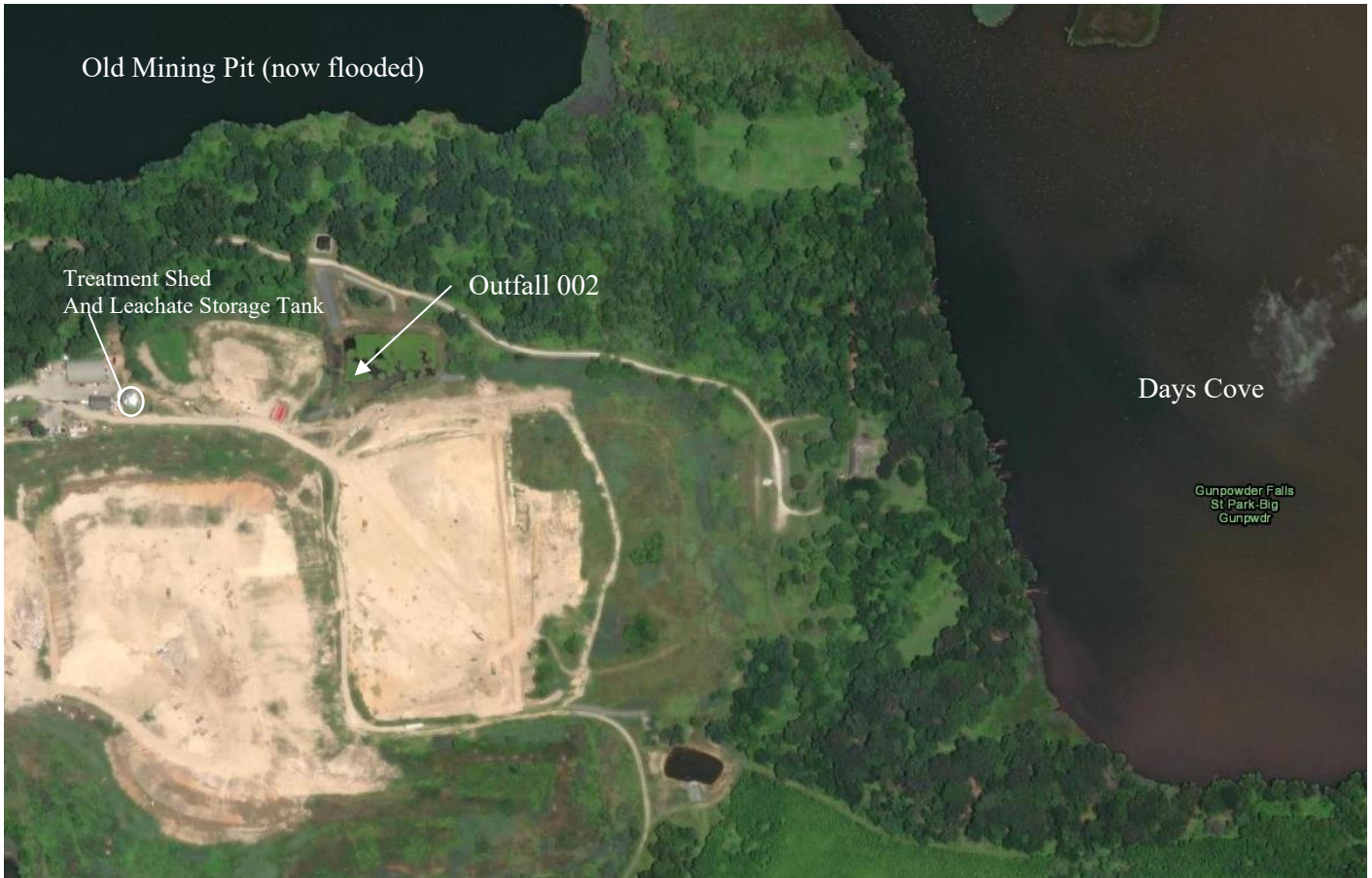
Figure 1. Days Cove Rubble Landfill and Days Cove
