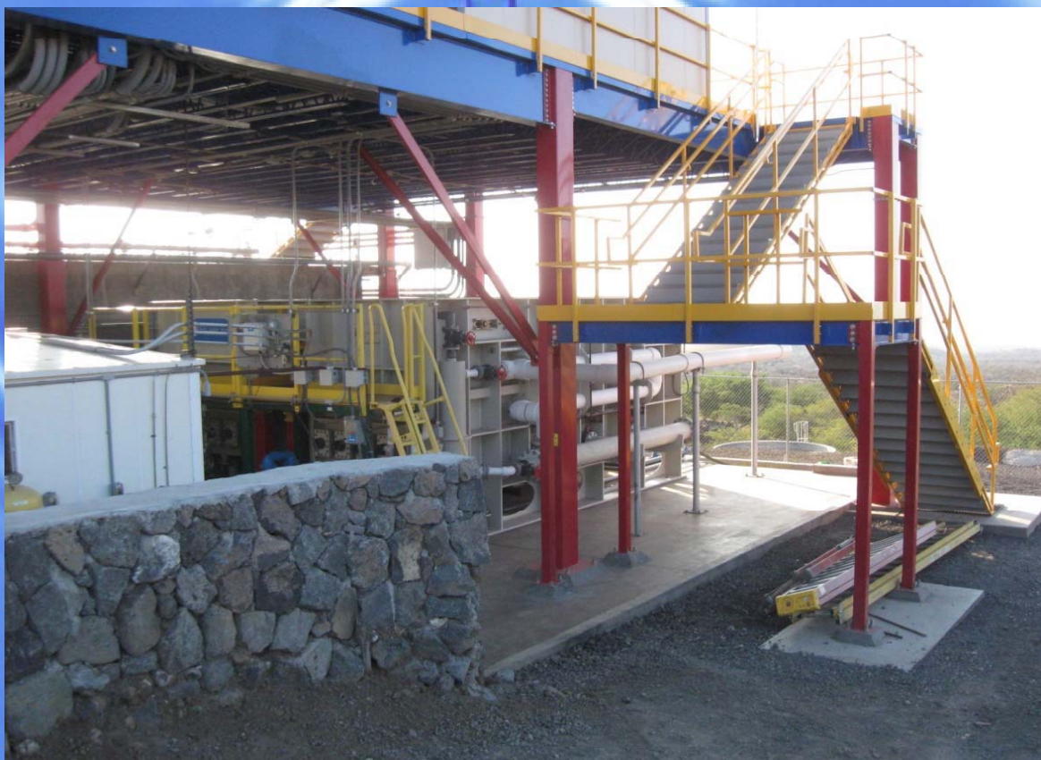
Lower Process Area & Side view of Upper Mezzanine
