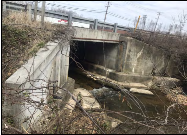
Middle blockage at Pulaski HWY (US 40) culvert
