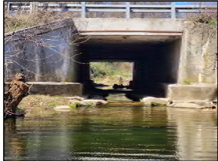
Middle blockage at Pulaski HWY (US 40) culvert
