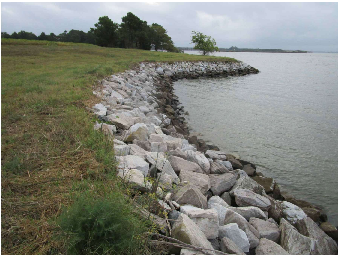
EXISTING RIPRAP PHOTO TAKEN BY LANE ENGINEERING, LLC 09/17/2024
