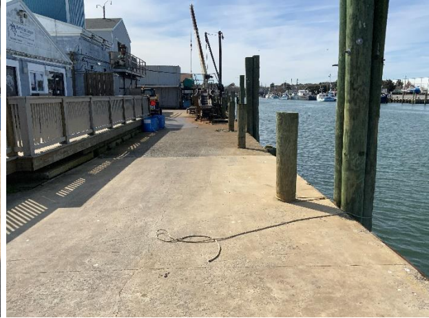
Photo 2: Overall view of fixed wharf deck from Station 1+60 looking west.
