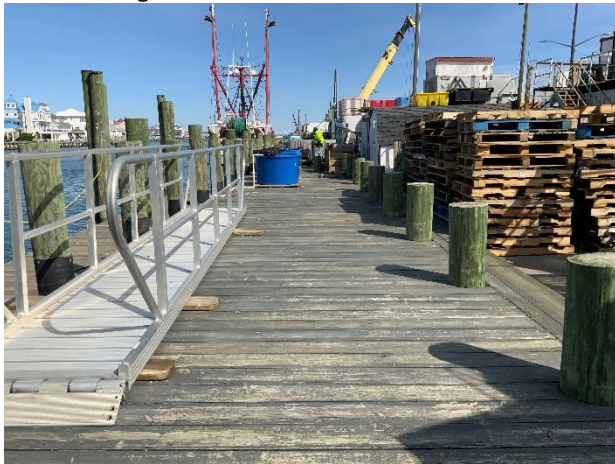
Photo 3: Overall view of fixed wharf deck from Station 1+79 looking east.
