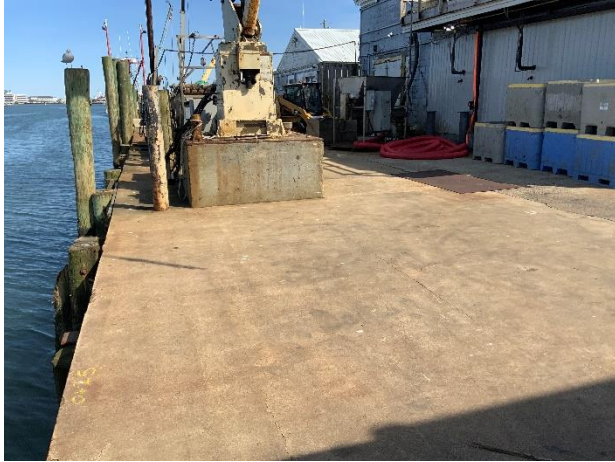
Photo 1: Overall view of fixed wharf deck from Station 0+00 looking east.
