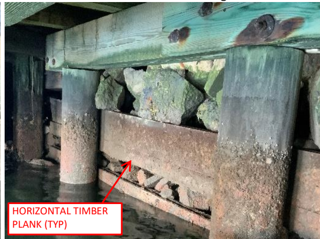
Photo 10: Underdeck view of bulkhead segment B.
