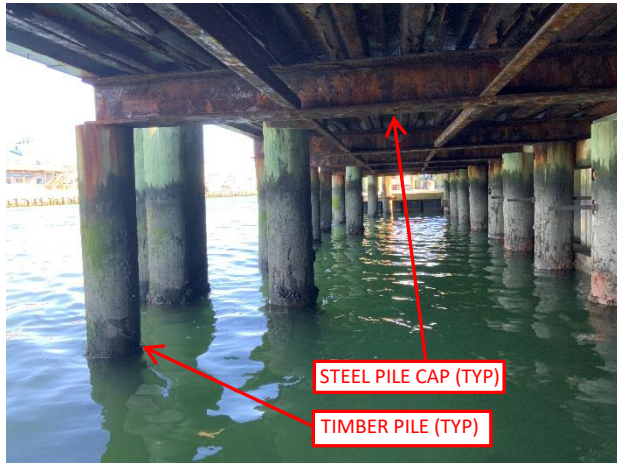
Photo 7: Underdeck view of wharf segment C.
