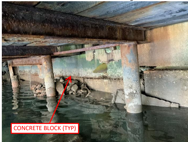
Photo 9: Underdeck view of bulkhead segment A.
