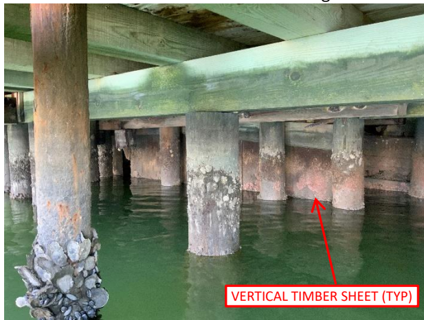
Photo 11: Underdeck view of bulkhead segment C.
