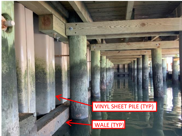
Photo 14: Underdeck view of bulkhead segment E, beneath wharf segment D.
