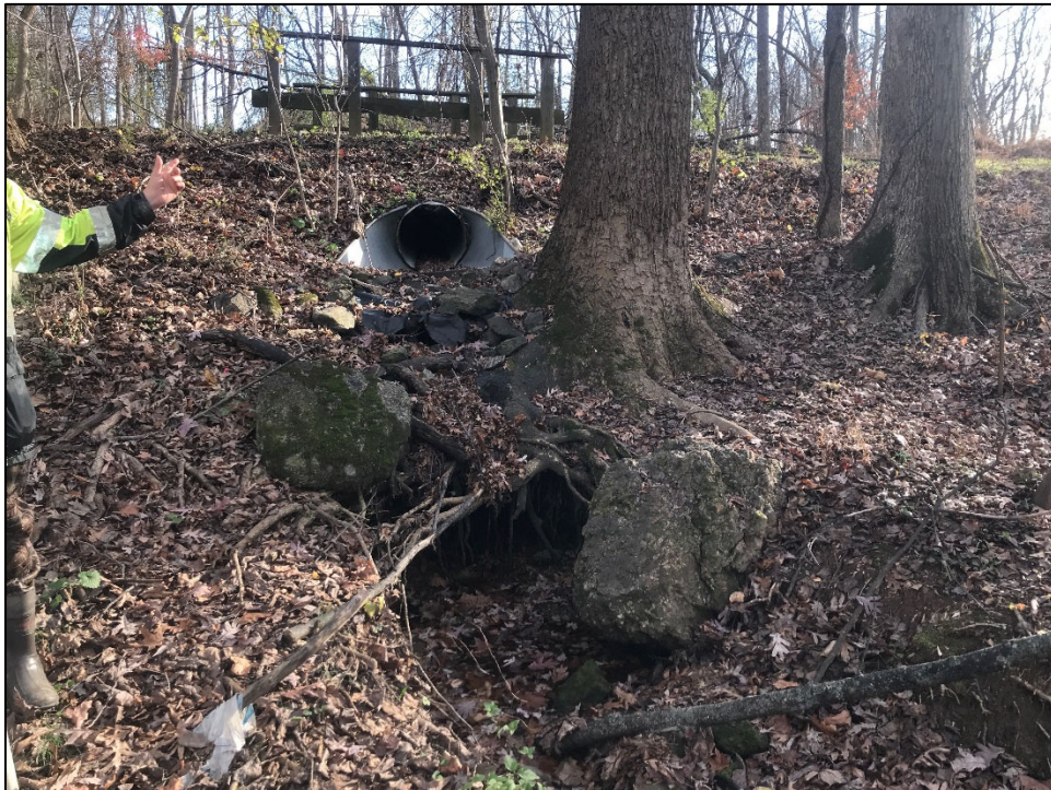
Photo 20: Reach 15-2, looking upstream near culvert under a pedestrian path, 2' head cut that is beginning to undercut a tree.
