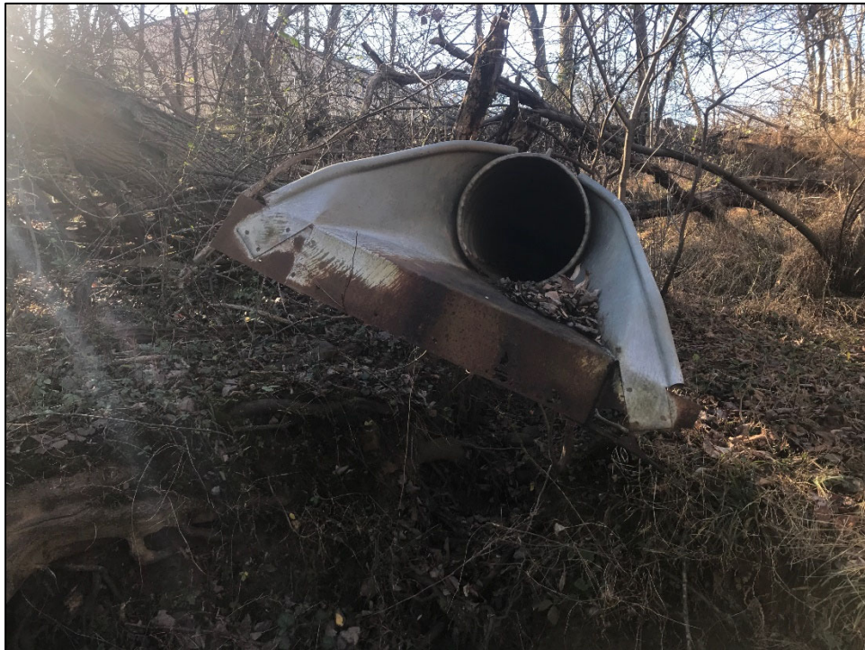
Photo 26: Reach 17, looking at outfall near Dobin Rd, the pipe has broken and is disconnected from the reach.
