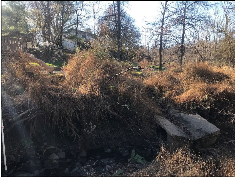
Photo 29: Reach 21A, looking at concrete swale near DeerPasture Dr, swale is disconnected from the stream and near failure.
