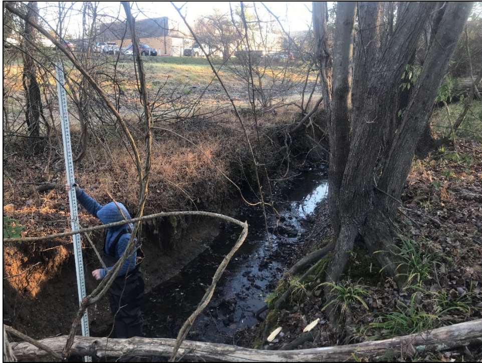
Photo 25: Reach 16, looking upstream near the confluence with Reach 15A, 4' eroding banks with minimal riparian vegetation.
