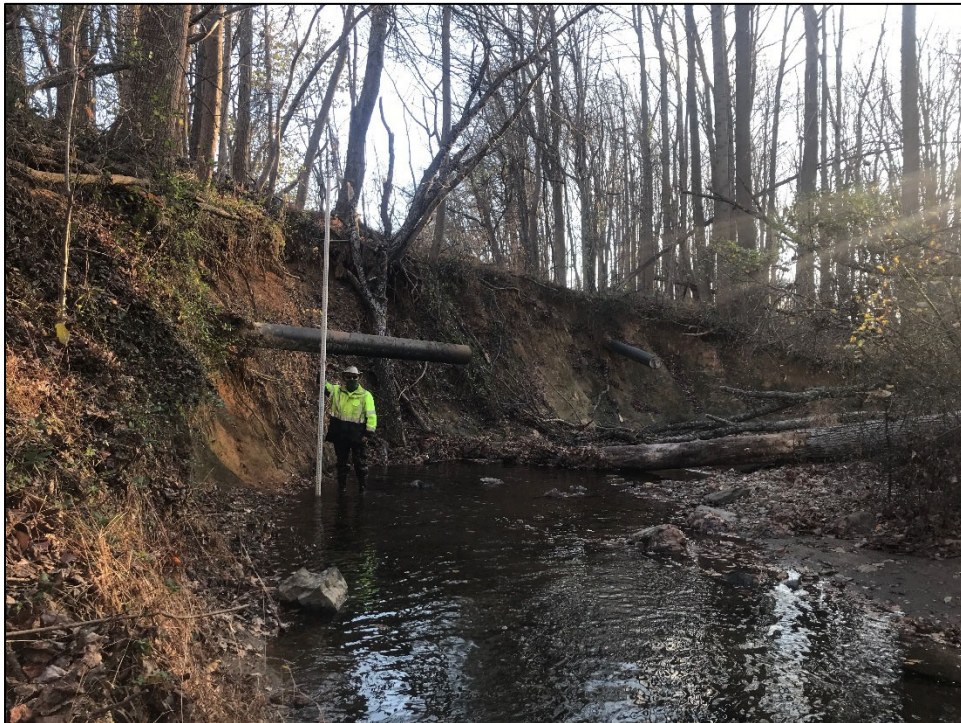
Photo 12: Reach 8B, looking downstream near Route 175, 12' actively eroding bank with disconnected and exposed pipes.
