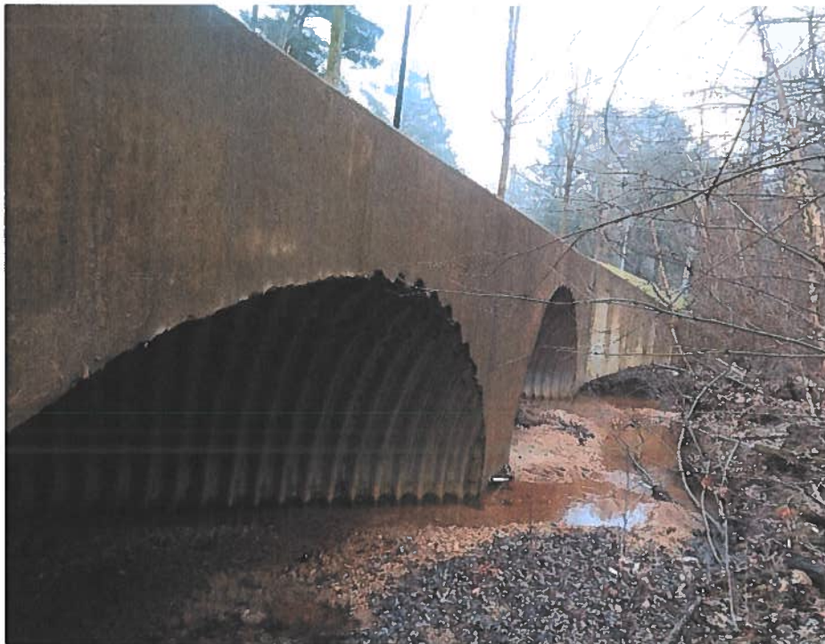
Pipe arch culvert at Four Seasons Drive (downstream)
