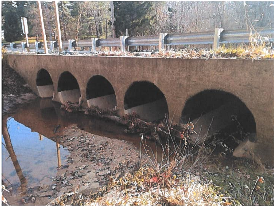
a) Circular culvert at Route 7 (upstream)
