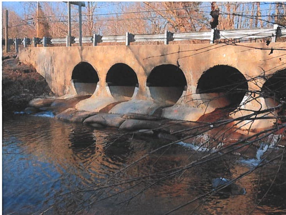
b) Circular culvert at Route 7 (downstream)
