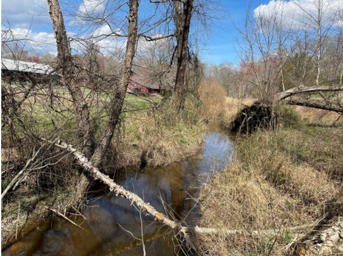
Photo 4: Downstream view of SR-3, note lack of distinct facet features and high banks indicating disconnection from floodplain.
