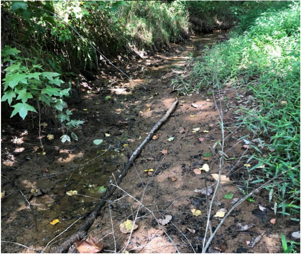
Photo 13: Upstream view on SR-2, note dewatering of stream channel and undercutting of right bank.
