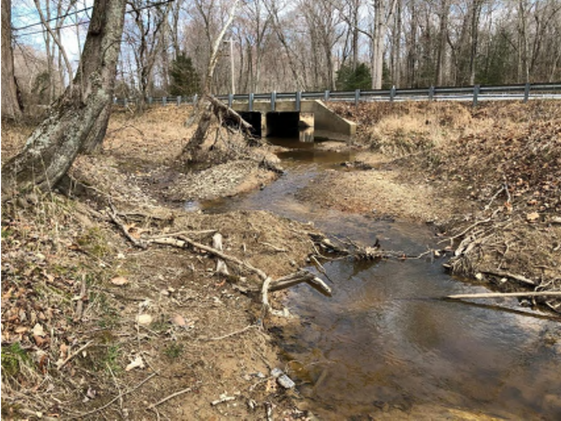
Photo 9: Upstream view of SR-1 at Marshall Hall Rd.
