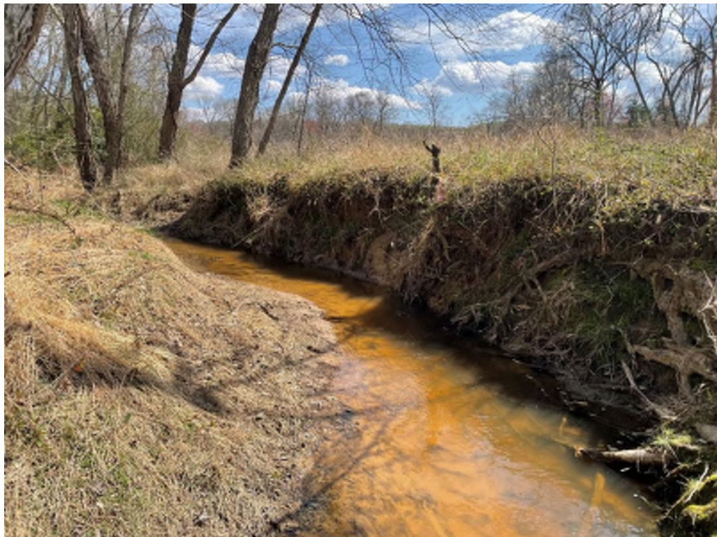
Photo 2: Upstream view of high cut banks of SR-3 consisting of a thick legacy sediment layer indicating disconnection from floodplain.
