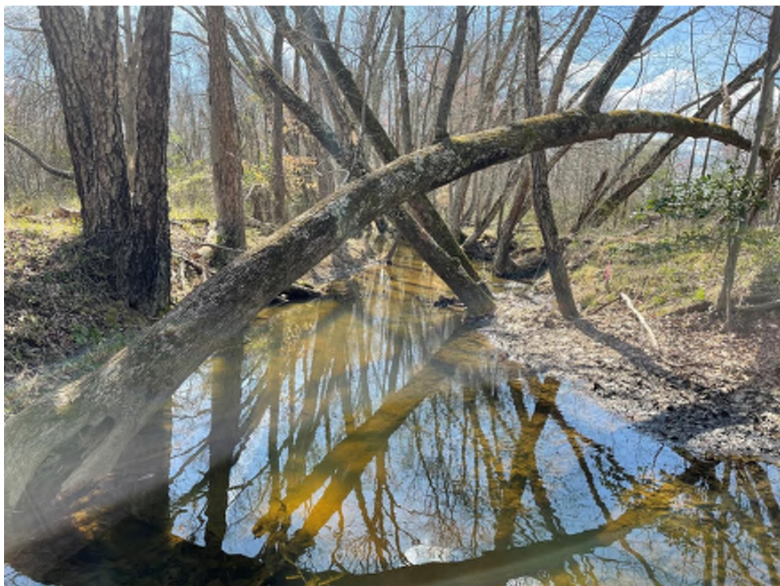
Photo 6: Downstream view of SR-4, note trees collapsing into stream channel typical within reach.
