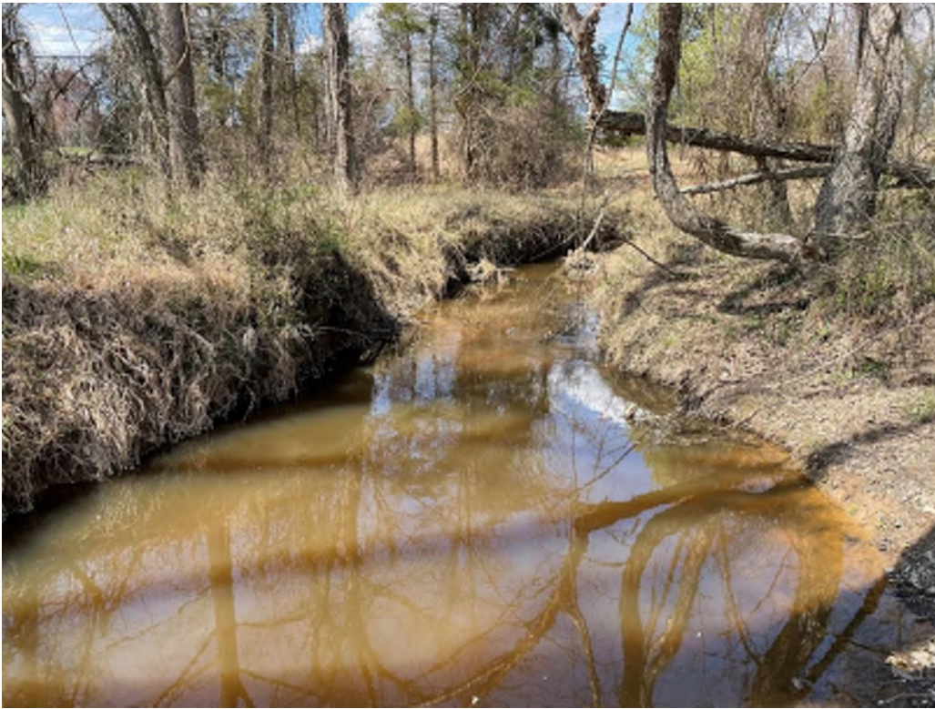
Photo 1: Downstream view of Mill Swamp on SR-3, note high, undercutting left bank.
