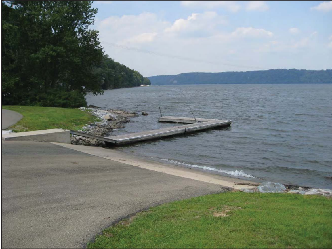
Figure 5.1.5-1: Boat Ramp and Dock
