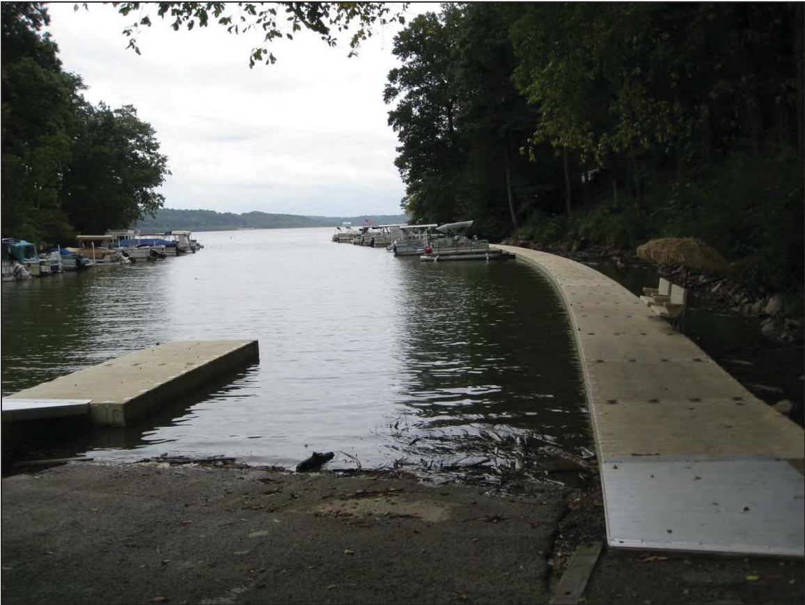
Figure 5.1.10-1: Glen Cove Marina Launch and Slips
