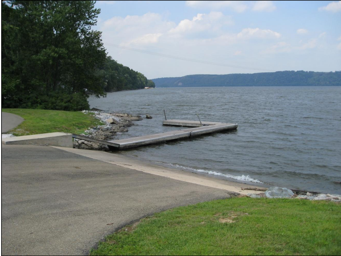
Figure 5.1.5-1: Boat Ramp and Dock
