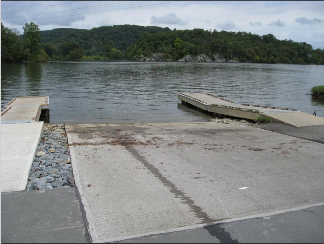
Figure 5.1.3-1: Muddy Creek Boat Launch
