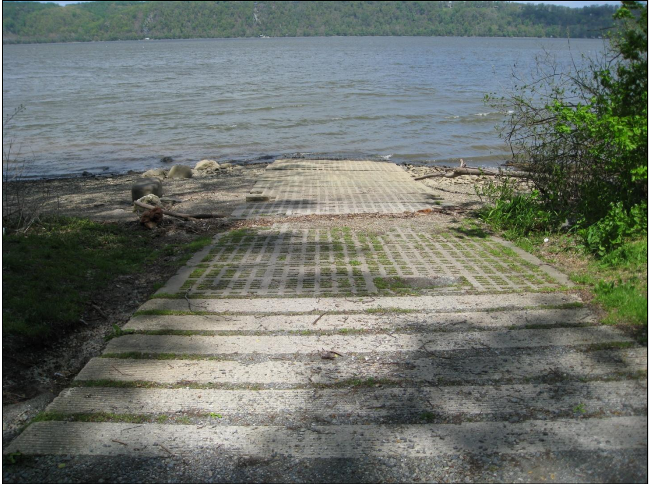
Figure 5.1.4-1: Cold Cabin Boat Launch
