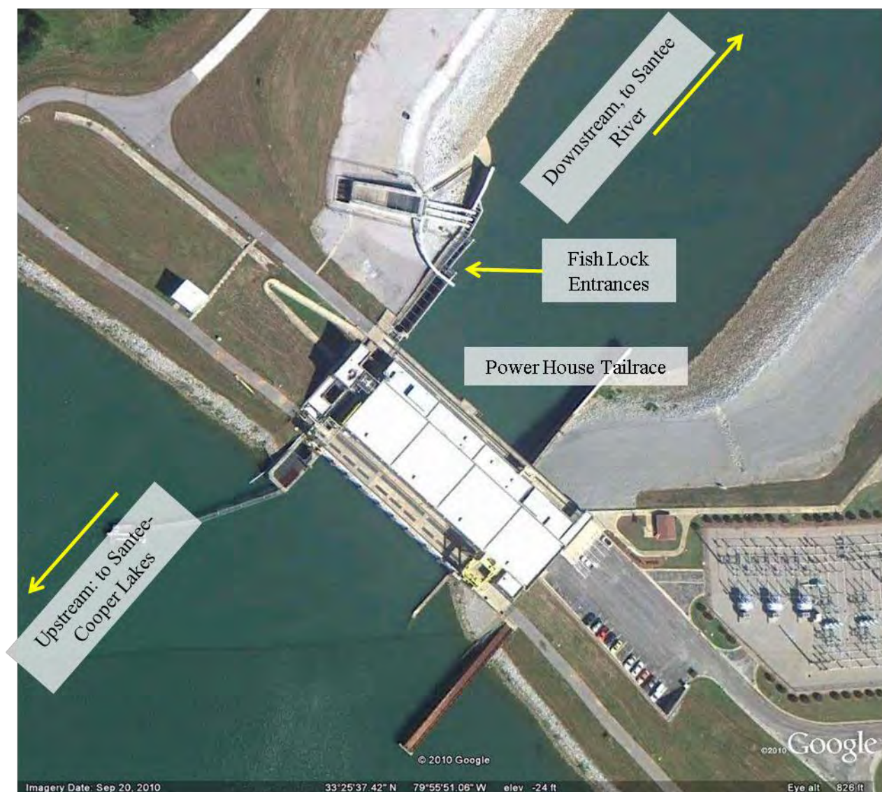
FIGURE 2.6-6: AERIAL IMAGE OF ST. STEPHEN DAM, REDIVERSION CANAL, SOUTH CAROLINA.
