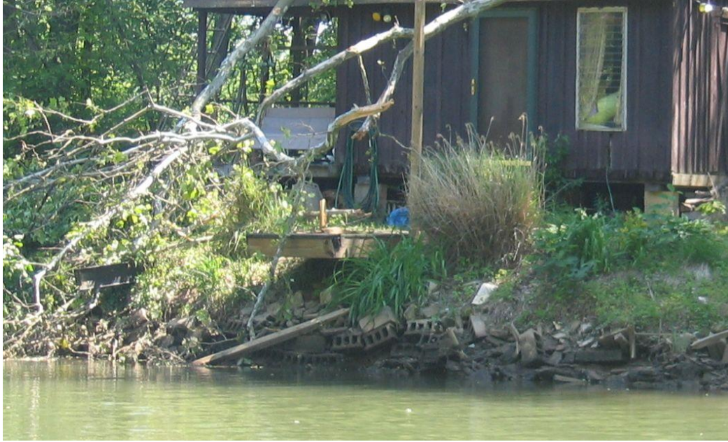
FIGURE 4.1.2-3: COLLAPSING CINDER BLOCK BULKHEAD (MAY 2008)
