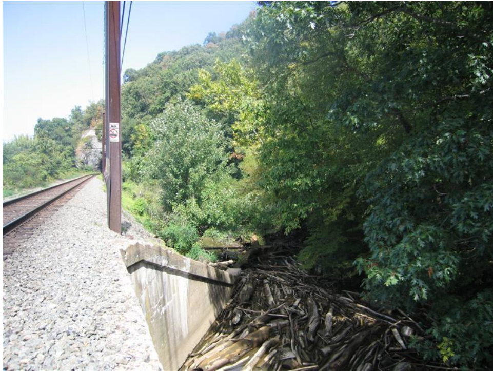
FIGURE 4.1.1-7: DEBRIS BUILD-UP AT TRIBUTARY CULVERT (SEPTEMBER 2007)
