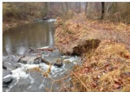
Outflanking of Instream Structures
