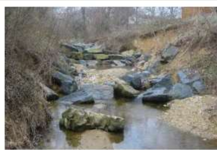
Bank Armoring Collapse
