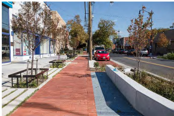
The Kennedy Street revitalization project in northwest Washington added more than 13,000 square feet of green space to a city block. It will help reduce combined sewer overflows into nearby Rock Creek Park during major rainfall events.
