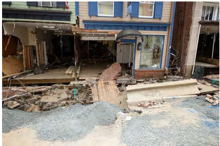
Flood damage along Main Street in Ellicott City on August 10, 2016. The suburban developments that have sprung up all around the town over the last 50 years have heightened flood risk during storm events by preventing natural drainage.
