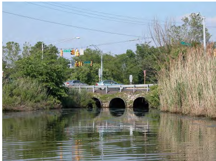
Stormwater culverts discharge into a marsh along Maryland's Avon River, which empties into the Chesapeake Bay.
