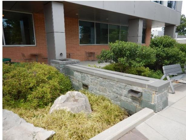
*Bioretention and rooftop disconnect are designed to complement the architecture*
