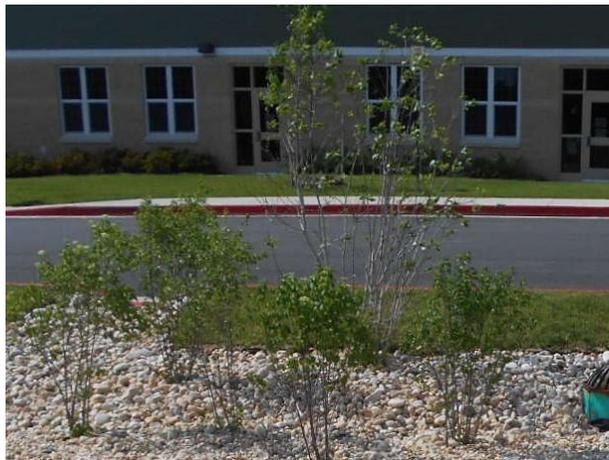
*Stone prevents weed growth and erosion in this bioretention*
