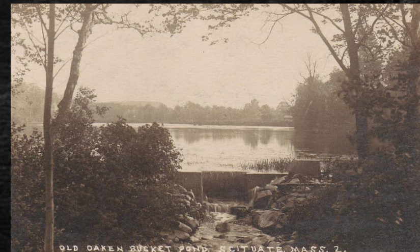
Old Oaken Bucket Pond Dam
