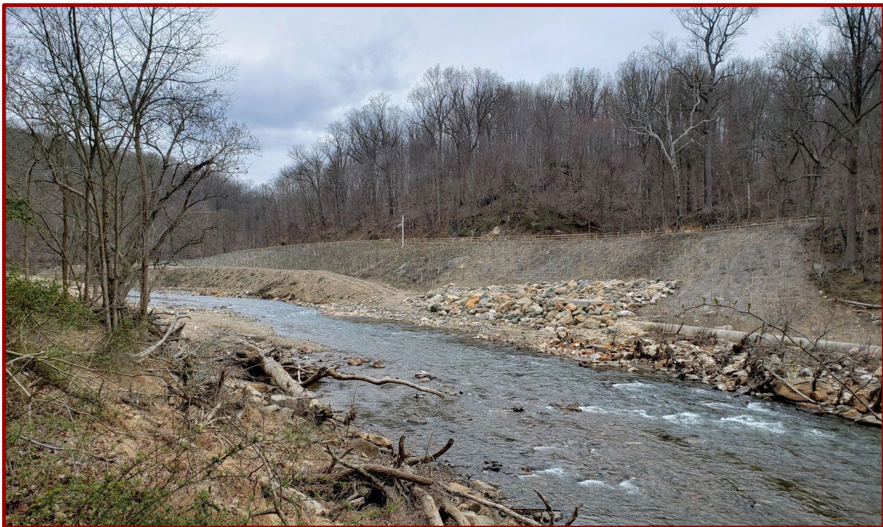
Figure 6.1: Former Bloede Dam site on the Patapsco River. Approximately 60 miles of habitat, including the mainstem and tributaries, are now open to migratory and resident fish post removal.
