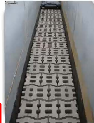
CSU Flume (Note 1-1/2 Blocks)
