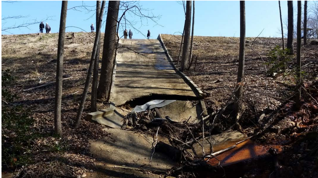
Figure 3-2.—Concrete delamination due to thermal expansion (Reclamation, 1997).
