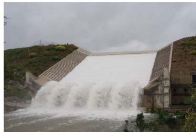
Figure Barriga-15.—Operation in May 2008 with estimated discharge of 350 - 530 ft 3 /s (courtesy of Morán and Toledo, 2006, all rights reserved).
