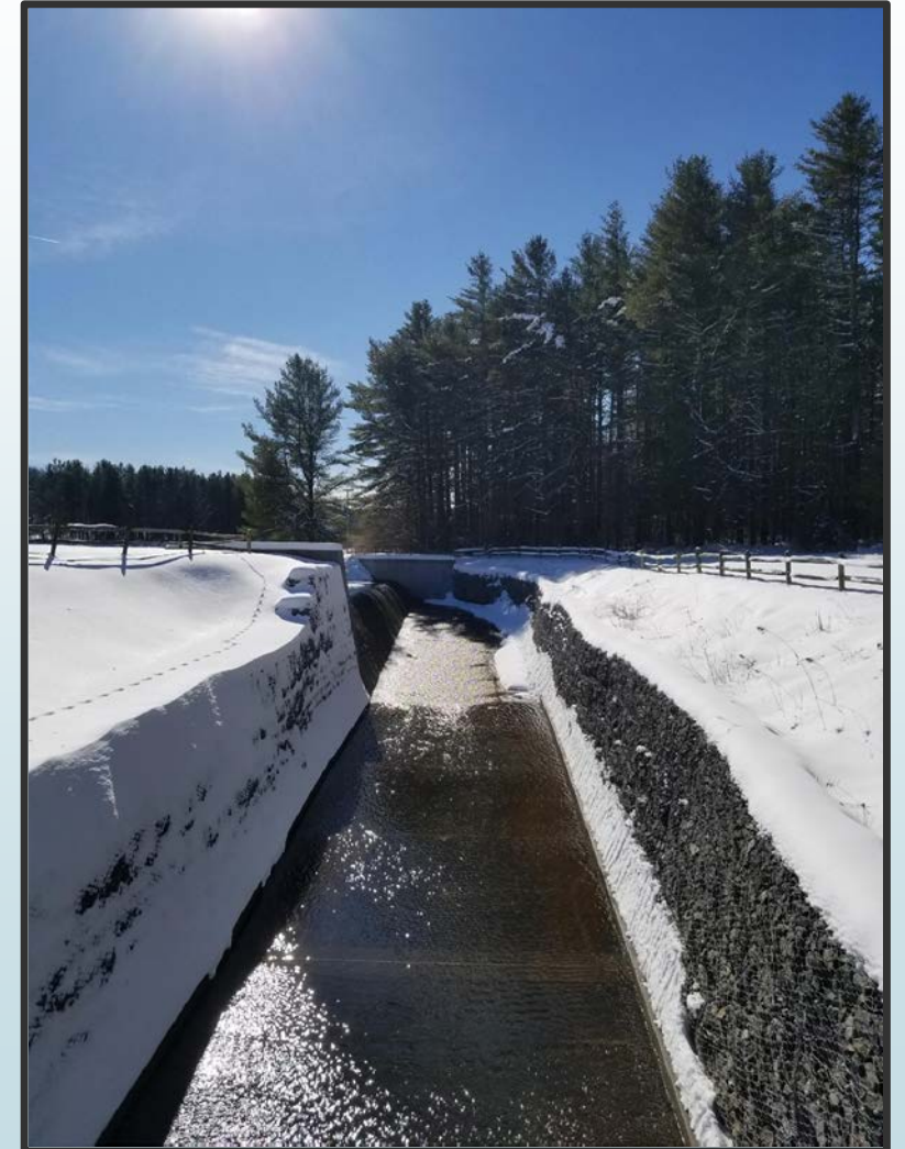
Harrington Manor Lake Spillway
