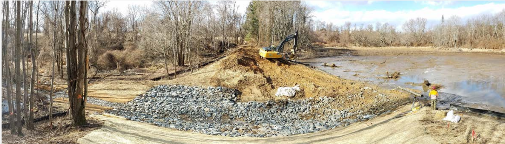
MDE File Photo: Martin Farm Dam. Harford County. Controlled Breach
