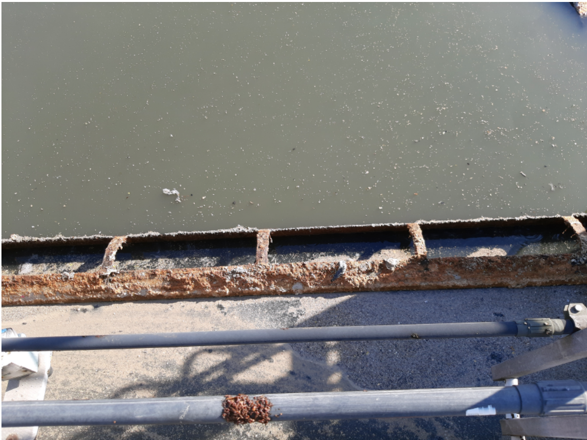
11/2/22 PST #1 – Note the heavy layer of scum and media on the surface of the water.
