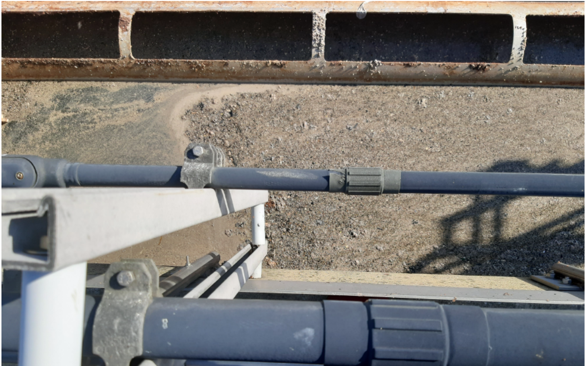
11/2/22 PST #1 – Note the heavy layer of scum and media on the surface of the water.
