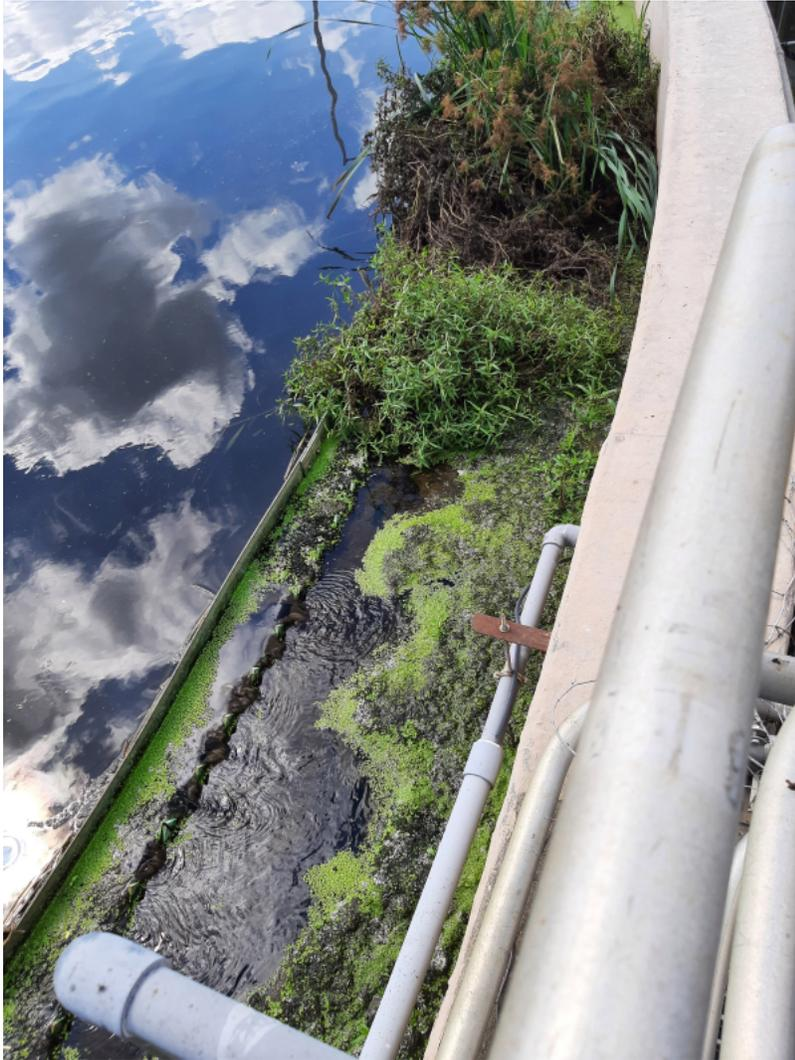
9/20/2021 Weir of secondary clarifier showing unacceptable blockage by algae and vegetative growth. This condition is impeding proper treatment process.
