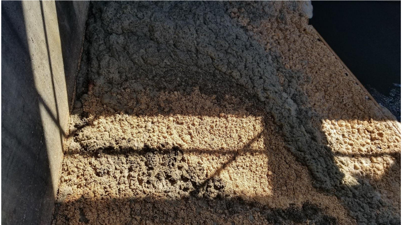
Figure 3b: Close up view of the FOGs comingled with media from the BAF cells. This floating FOG is also shown at the left side of the picture shown in Figure 3a.
