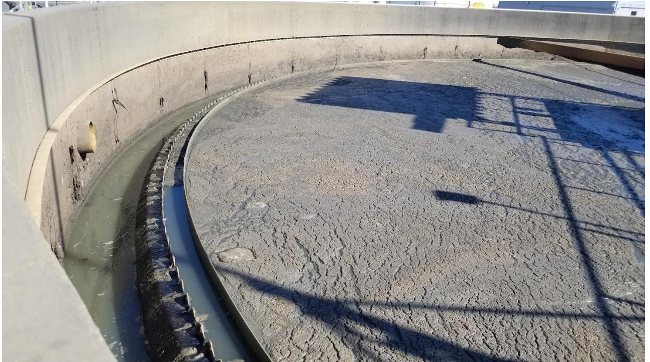
Figure 1a: Sludge next to the V- notch weir and on the surface of GST #1. The skimmer arm is above the water surface level.
