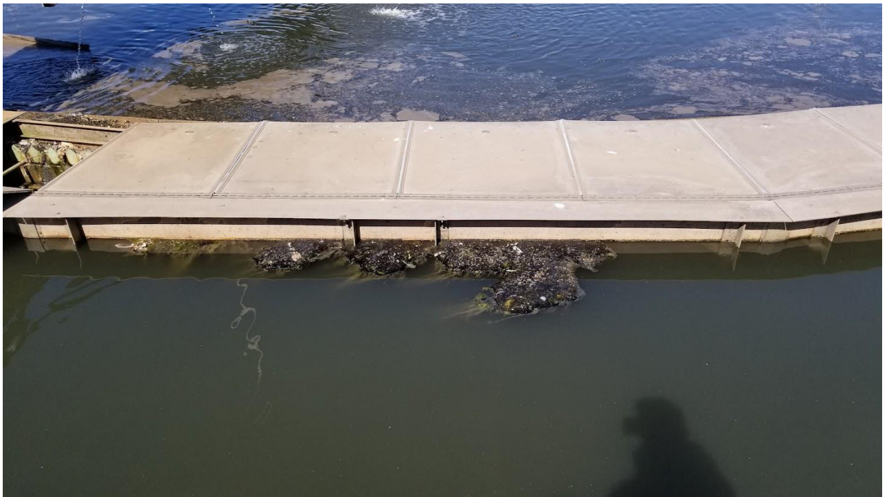
Figure 2b: Solids on the water surface in Clarifier #6A at two sides of the launder cover.
