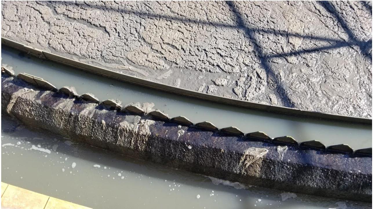
Figure 1c: Close up view of GST #1, with some rags stuck to the V- notch weir.
