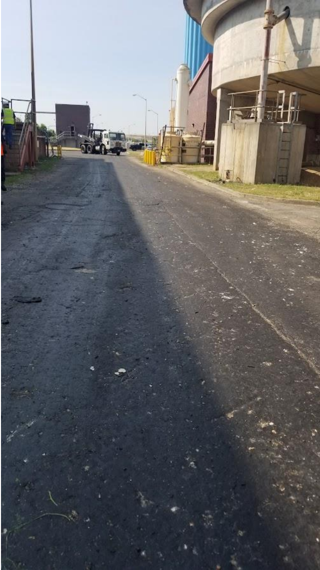
Figure 2c: Grease tracking and grit on the ground at the road west of the combined influent building. This picture was taken facing south.
