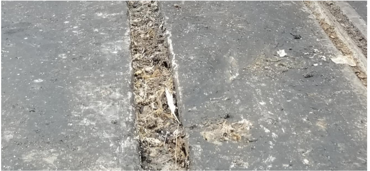
Figure 2e: Close up view of Figure 2d with some BAF media in the depressed area by the northwest side of the combined influent building.
