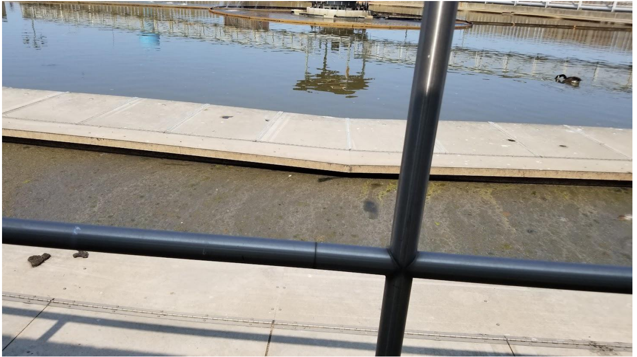
Figure 5c: Sludge between launder covers within Clarifier #4
