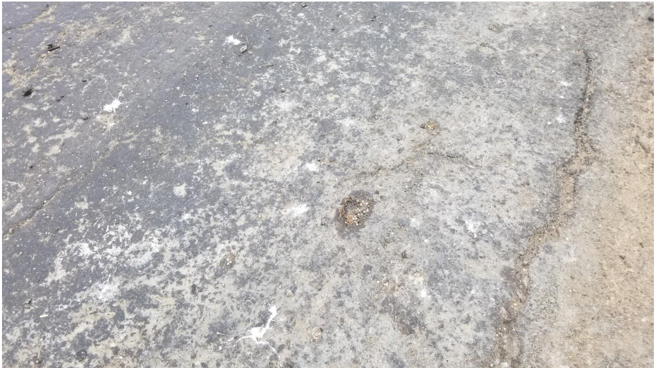
Figure 2f: Close up view of BAF media on the ground by the west side of the combined influent building and south of the area shown in Figure 2d.
