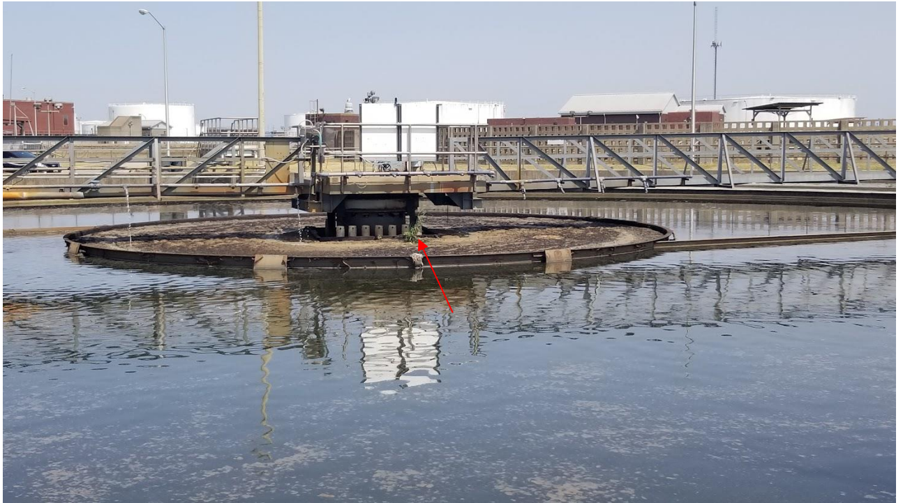
Figure 5m: Plant growing in the middle of Clarifier # 5A (pointed to with a red arrow).
