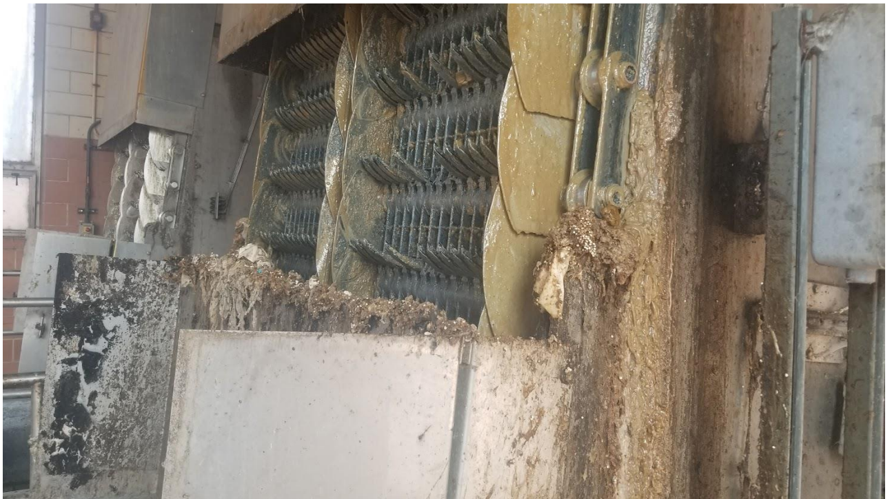
Figure 1a: BAF media on the side of bar screen #2.
