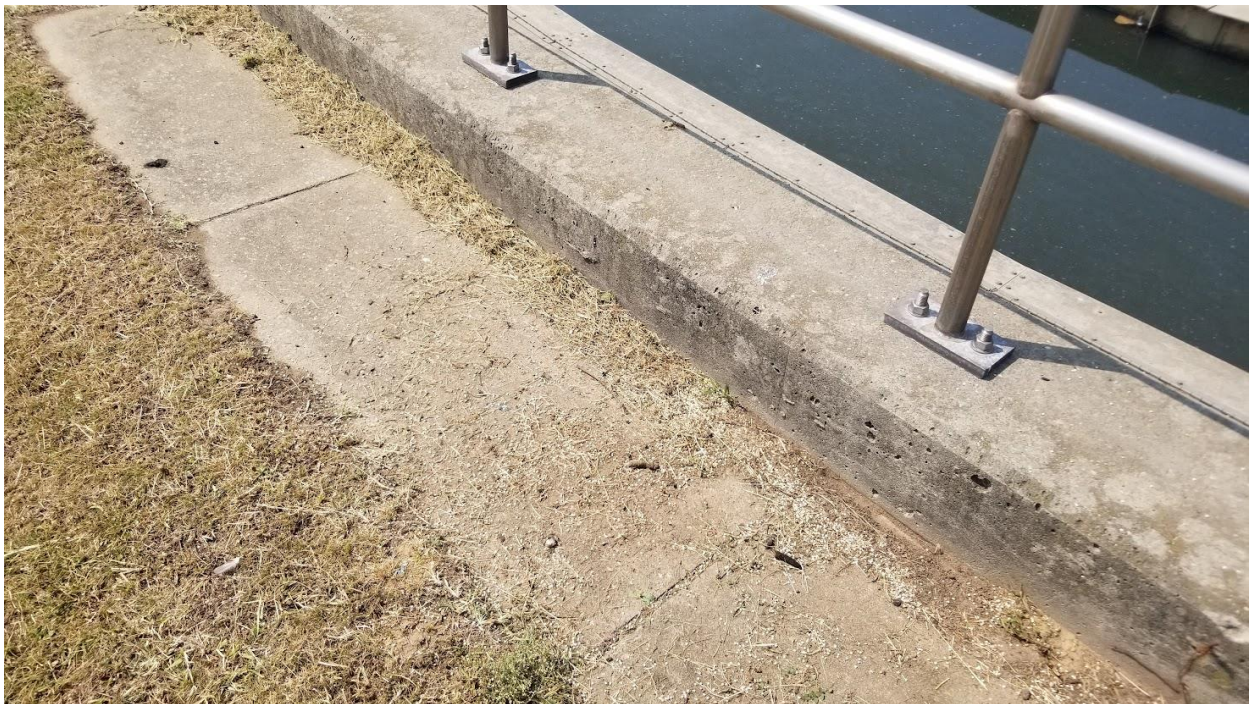
Figure 5h: Media on the ground by Clarifier #6B
