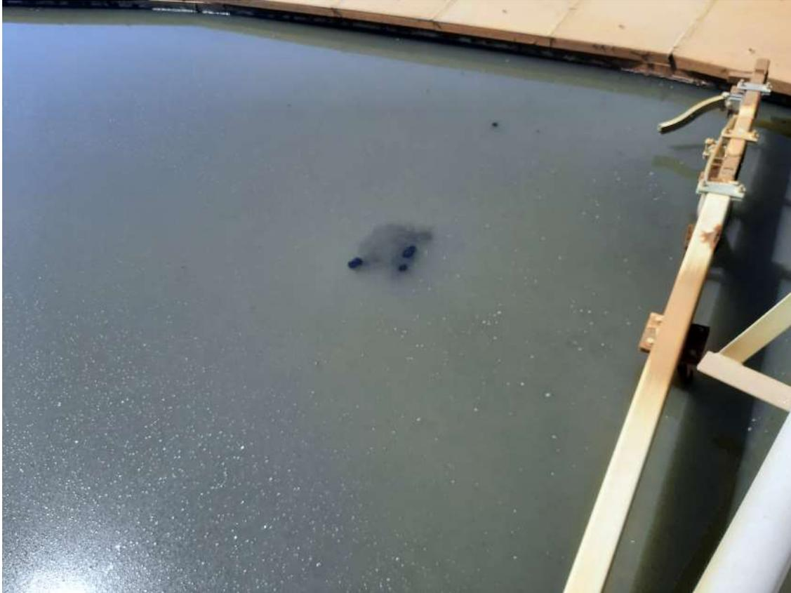
6/29/22 Secondary clarifier #4 methane gas bubbling from the surface and black balls of sludge floating on the surface
