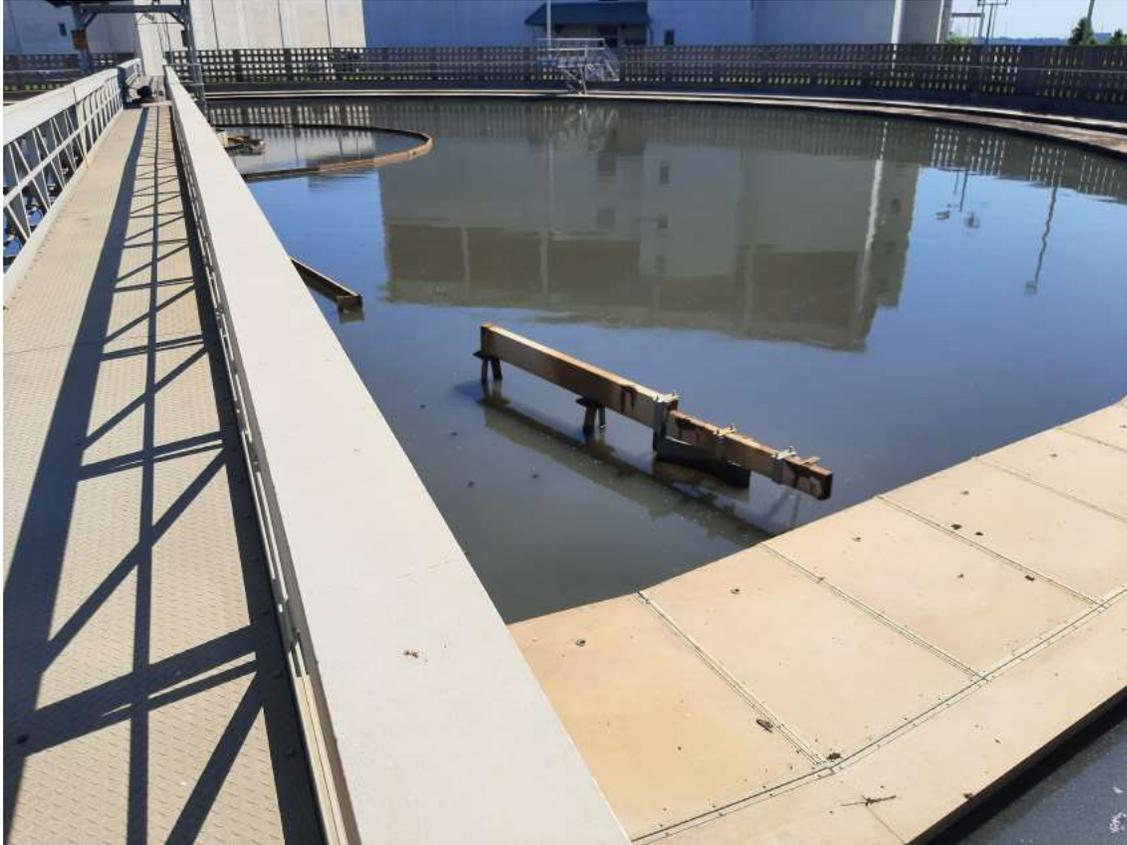
6/29/22 skimmer arm on clarifier #5A is slightly bent and the scum scraper is missing.
