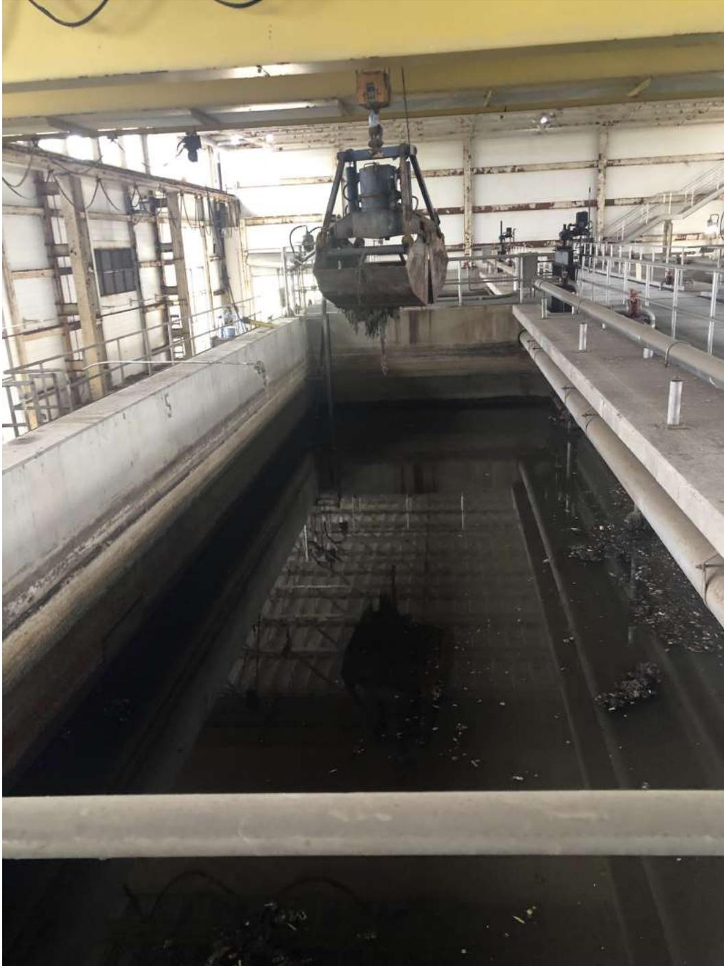
7/5/22 Grit tank and traveling crane with clamshell in Grit Building. Picture taken at my request by Hazen and Sawyer
