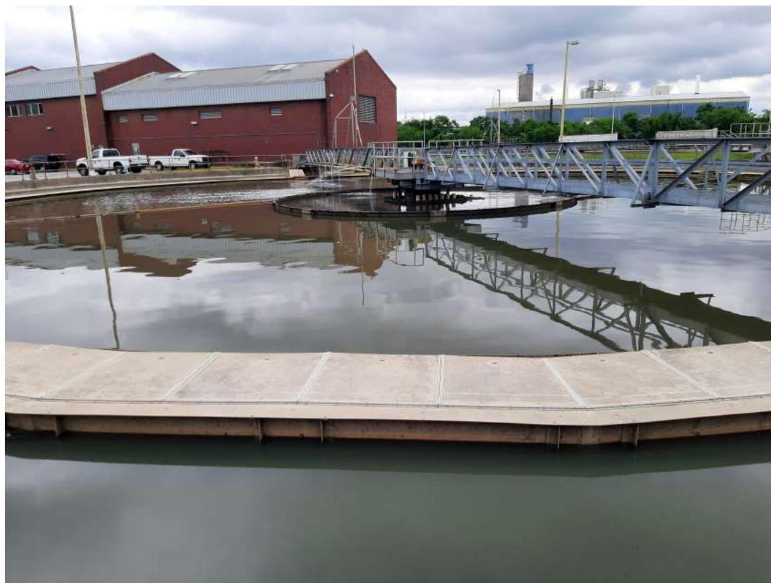
7/7/22 Secondary clarifier 6A RAS pump is functioning and the 6A clarifier is back in service
