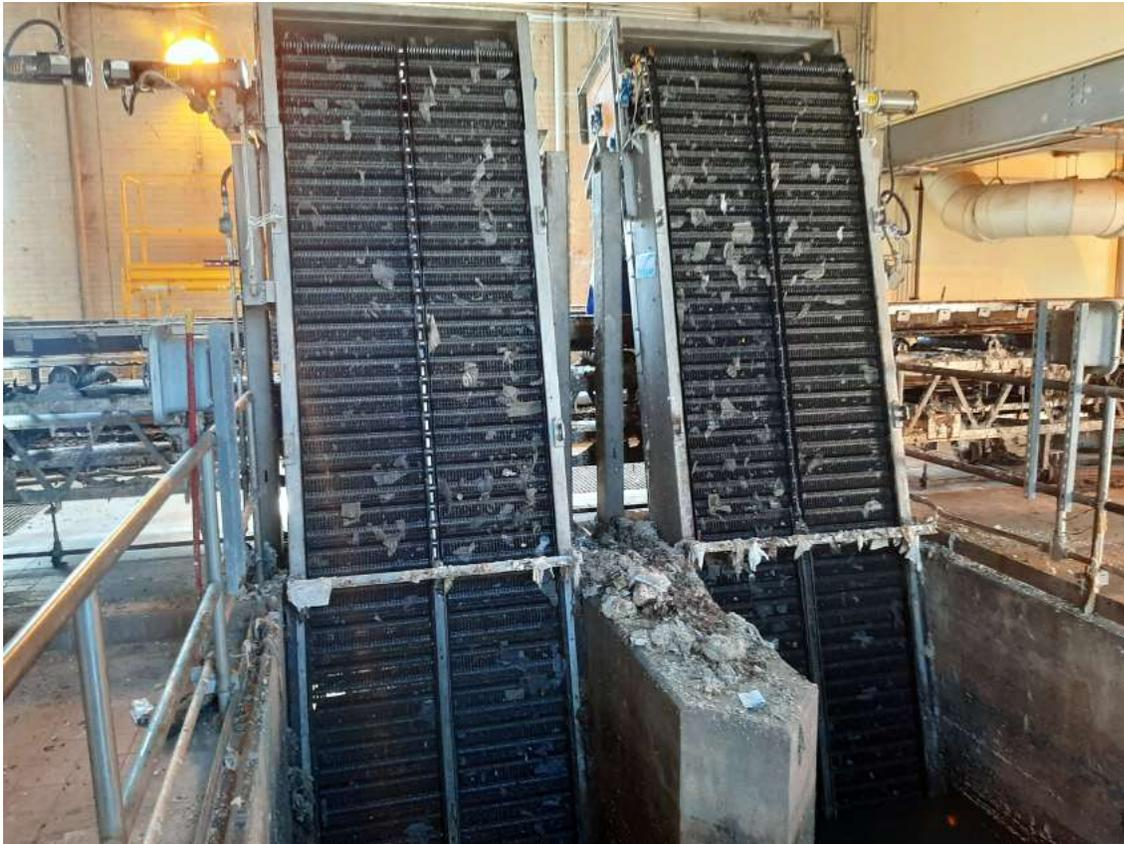
6/29/22 pile of trash from screening unit located in a position to get back into the system. The area should be checked and cleaned as appropriate.
