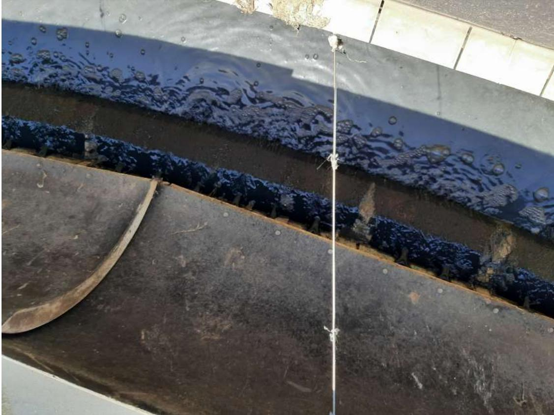
6/29/22 Effluent from GST #1 the weirs are blocked and covered with the sludge
