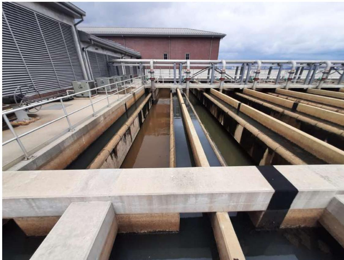
7/7/22 DNF taken offline and allowed to dry in an attempt to remove the algae on the overflow weirs
