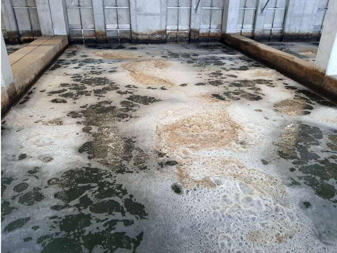
7/7/22 BAF filter cell – Note heavy foaming with solids
