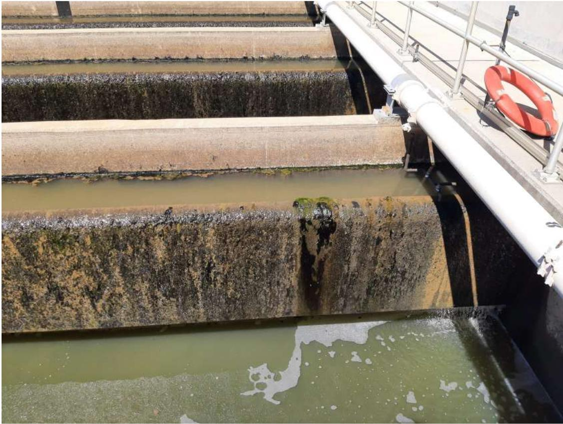
6/29/22 DNF filter cell – turbid water with floating scum
