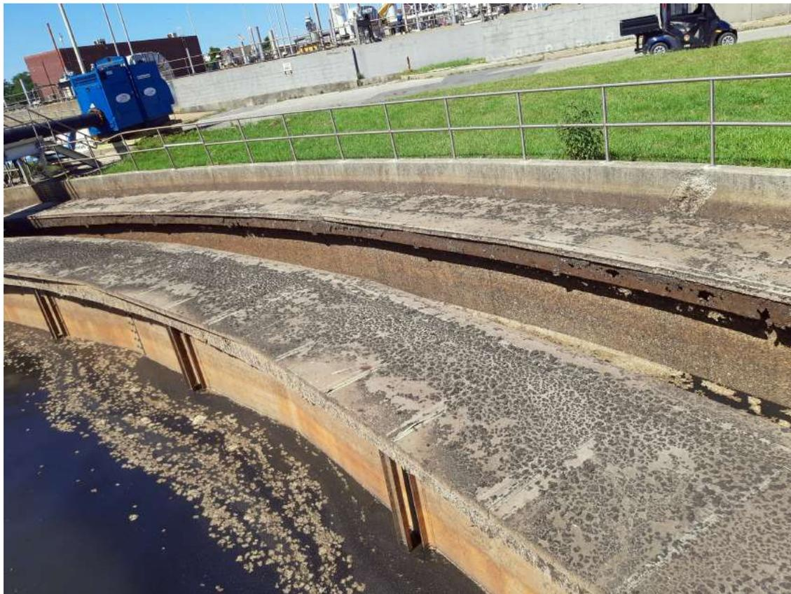
6/29/22 Secondary clarifier #3 is being used to collect the filter backwash discharge
