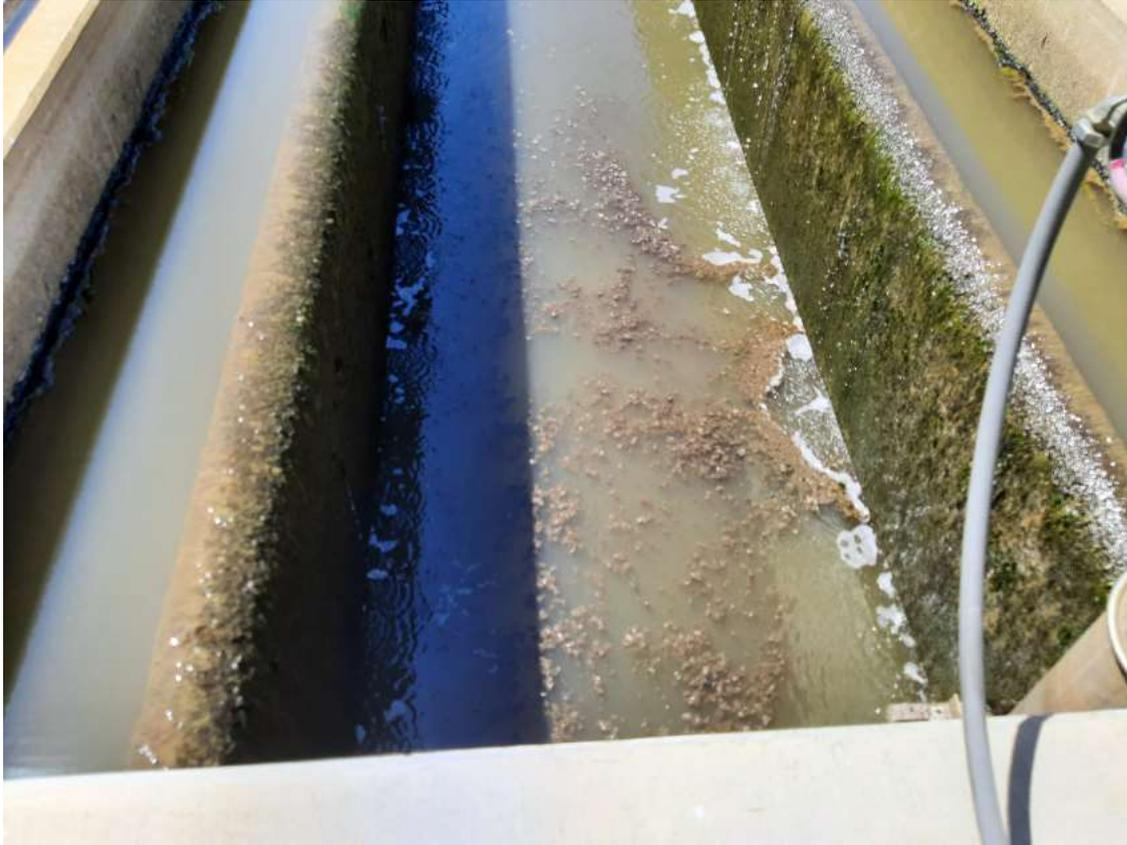
6/29/22 DNF – turbid water with floating solids
