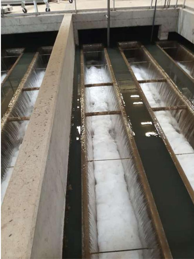
5/18/22 BAF effluent overflow cell Note excessive foaming caused by high BOD concentration
