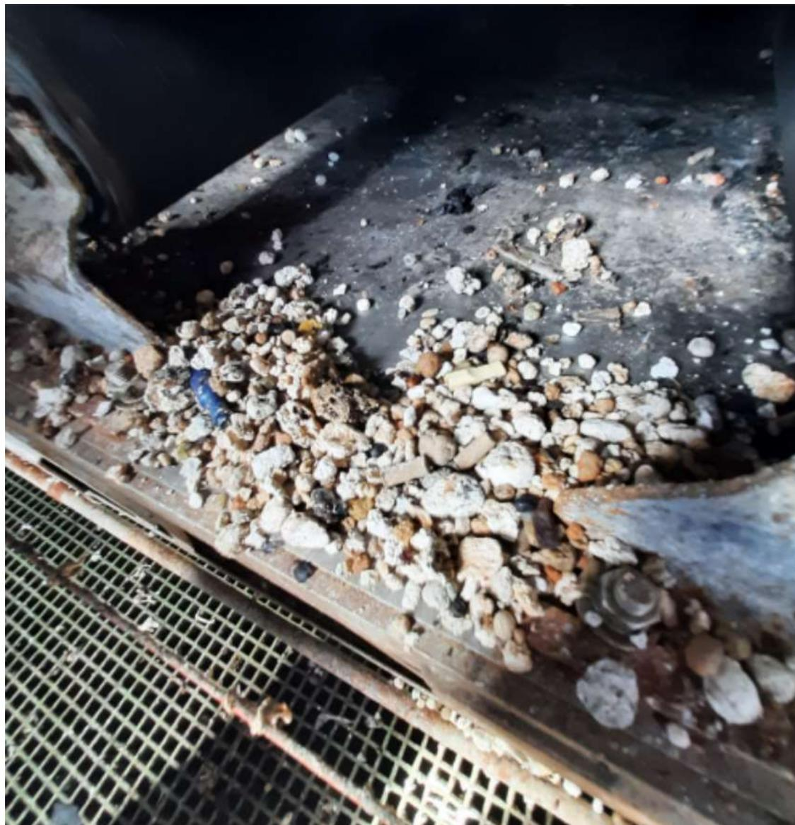
5/18/22 Trash and debris falling from the conveyor belts at the fine screening building
