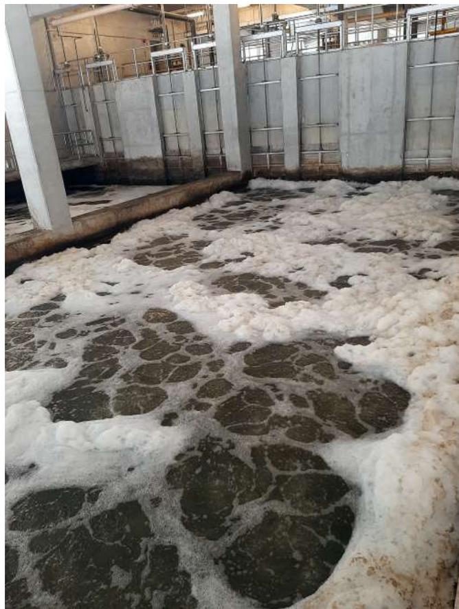
5/18/22 BAF filter cell Note excessive foam containing solids
