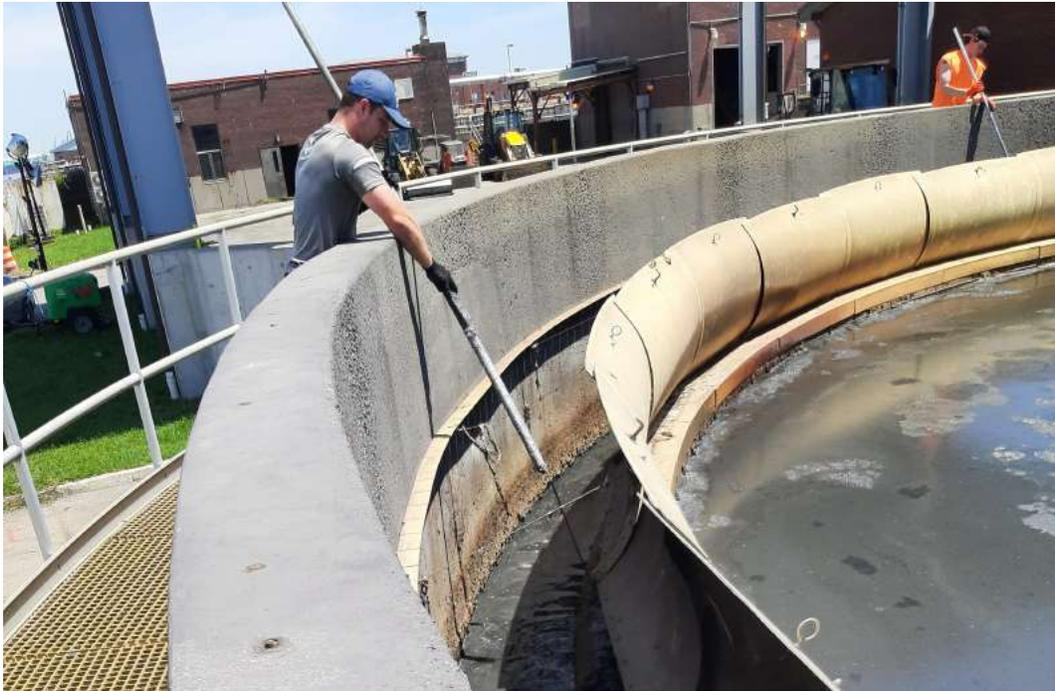
5/18/22 operators cleaning the solid particles that are accumulating on the weirs of the GST #1.
