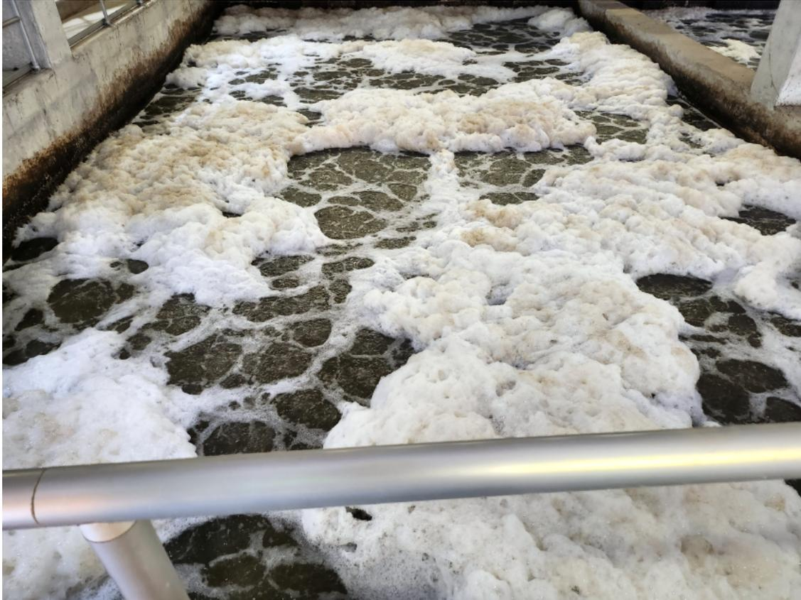
8/24/22 BAF cell. Note, excessive foaming.
