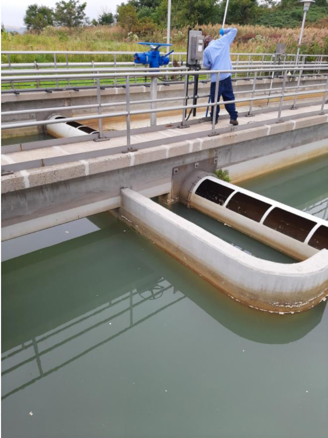
10/6/2021 operator manually skimming at the contact chamber
