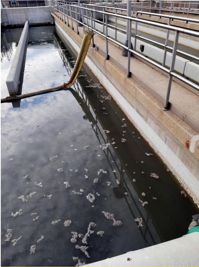
CCC – Dark grey turbid effluent with floating solids/ FOG traveling to scum log 1/31/22
