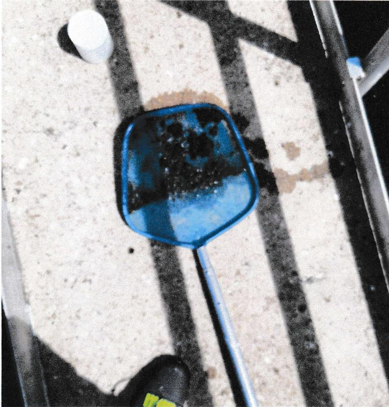
4/22/22 Floating solids skimmed from chlorine contact chamber
