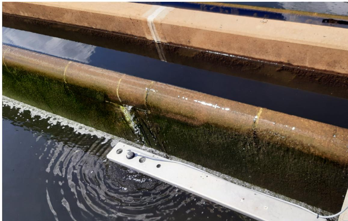
7/14/22 Water breach near the top of the weir
