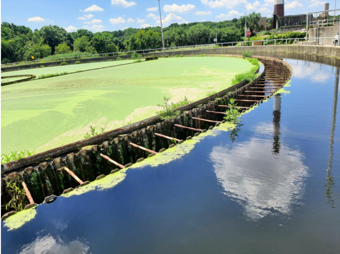
7/14/22 Blocked weirs due to algae and vegetation causing short circuiting of the weirs.
