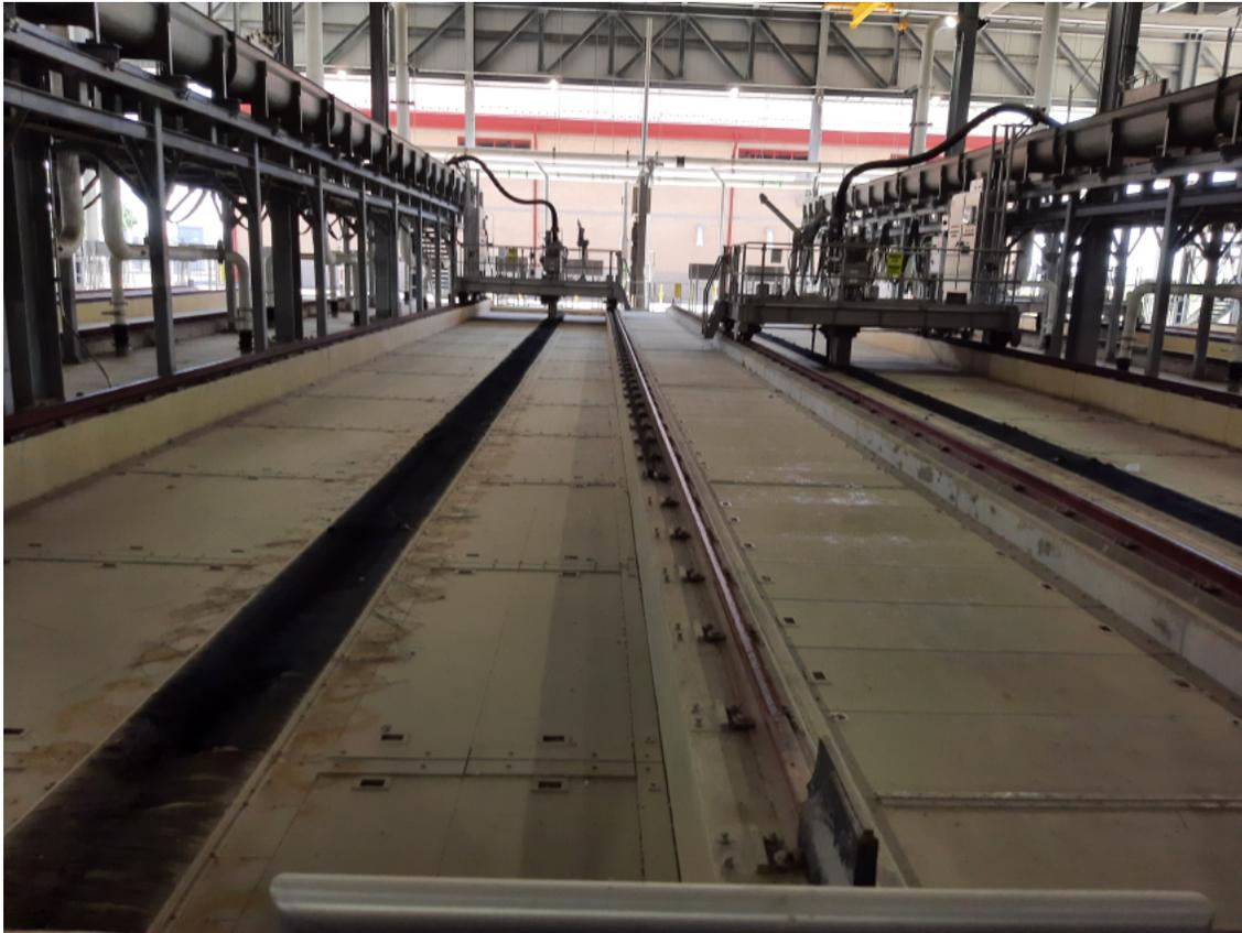
7/14/22 Grit removal system - Traveling Bridges suction the grit from the tanks to overhead conveyors that convey the grit to a dewatering system consisting of spinning classifiers.
