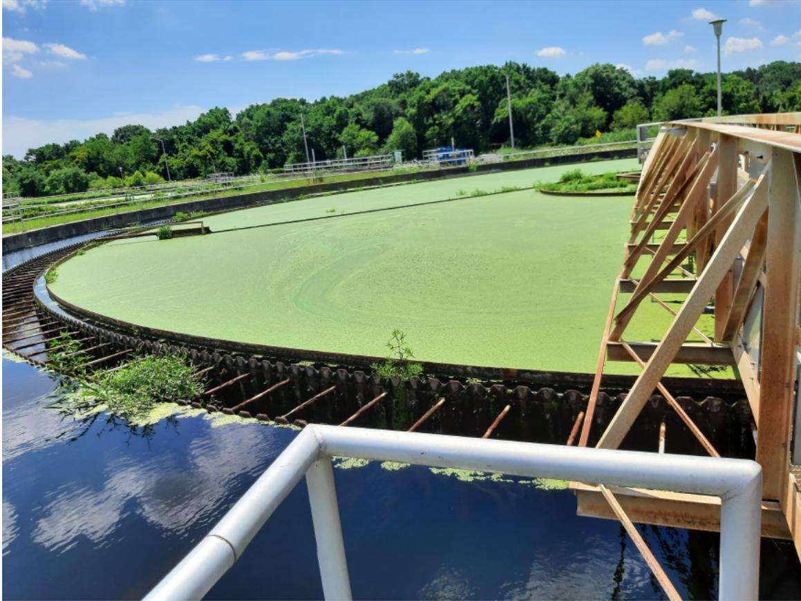
7/14/22 Vegetation and algae causing short circuiting of the weirs on the secondary clarifiers and large amounts of vegetation in the stilling well and floating on the surface of the water in the clarifiers.
