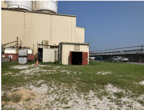
Image 04: Area outside the affected pit (pit is inside the double doors).
