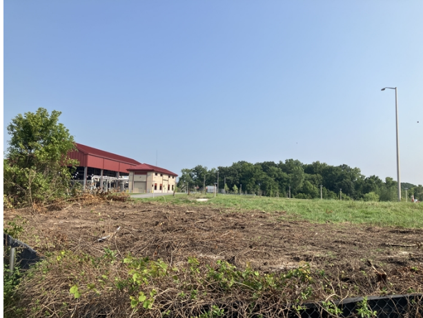
Image 07: Area downslope of cleanout, adjacent to lot.
