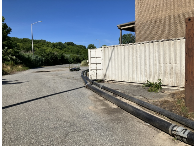
Image 05: Hose Split. Affected area in center of image.
