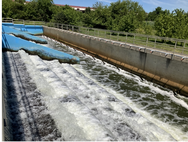
Image 04: Step Aeration system, final effluent.
