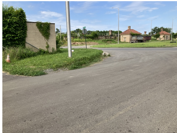
Image 07: Roadway and grassy area downslope from Stockpile pit.
