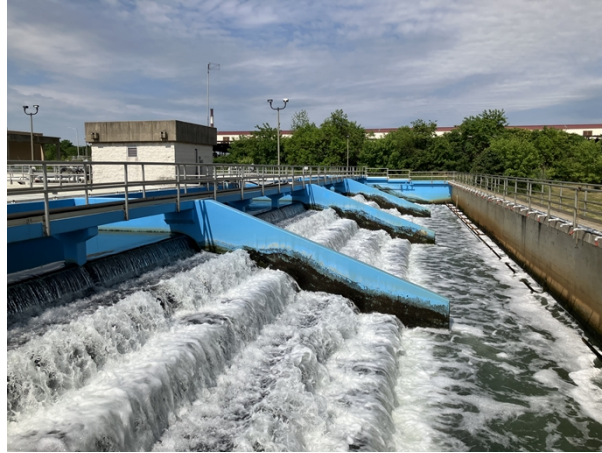
Image 02: Step Aeration system, final effluent.
