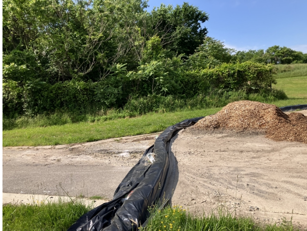
Image 04: New temporary berm.
