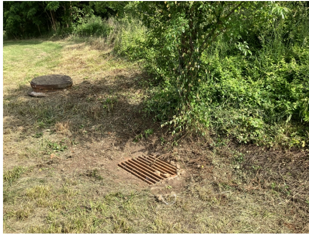
Image 03: Storm drain area clear.
