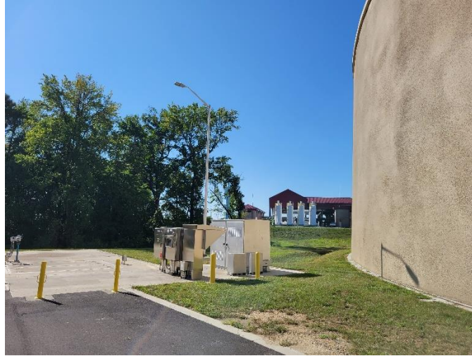
Image 8: Exterior, EQ Tank area.
