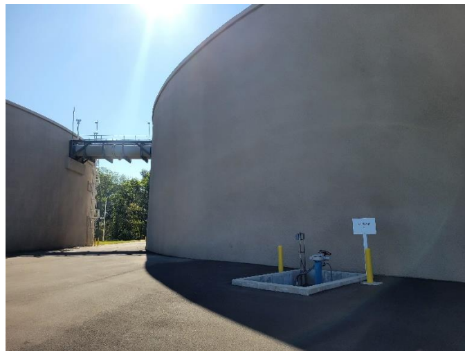
Image 7: Exterior, EQ Tank area.
