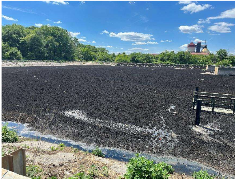
Sludge Storage Lagoon – West Side
