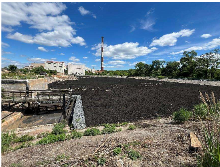
Sludge Storage Lagoon – East Side
