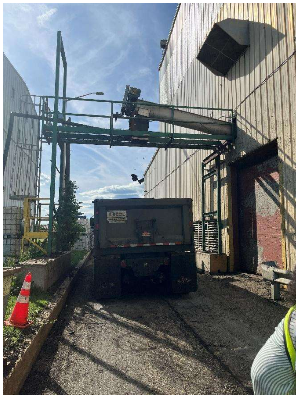
Dewatered Sludge Truck Loading
