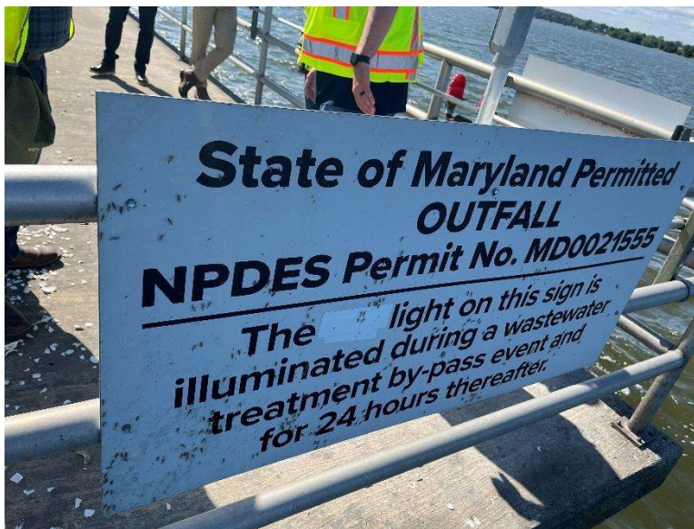
Outfall 001 Sign and Bypass Light Description
