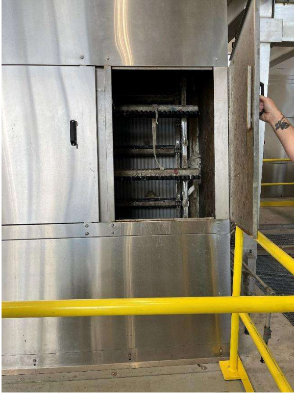
Coarse Screen Unit and Associated Dumpster
