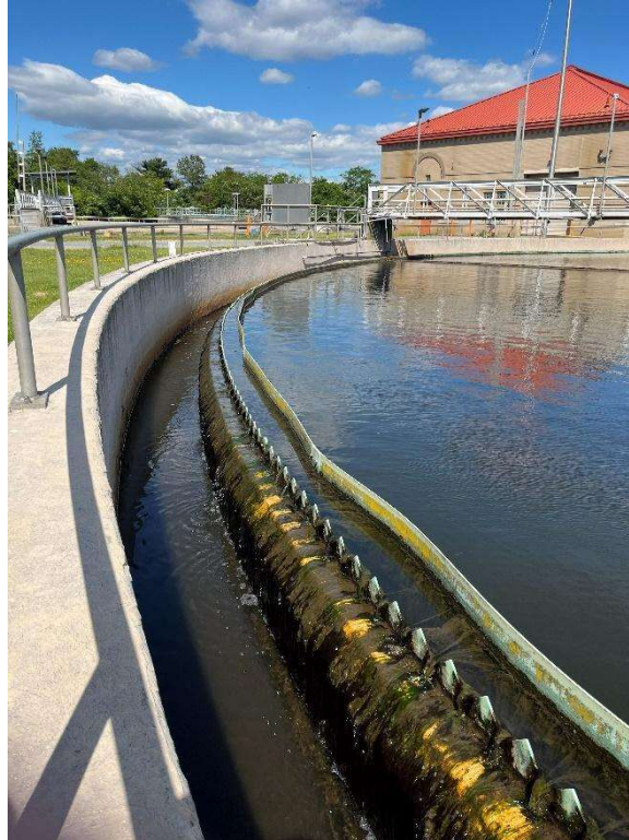
Secondary Clarifier Weir System
