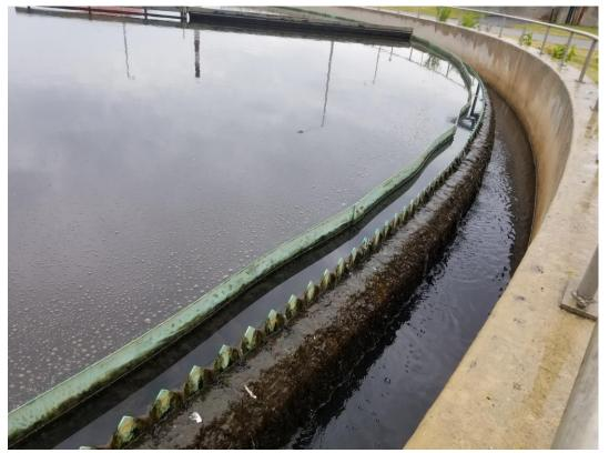
Picture 8: 6/14/23 – Secondary clarifier 5A was observed to have algae/vegetation growth along/past the weir.
