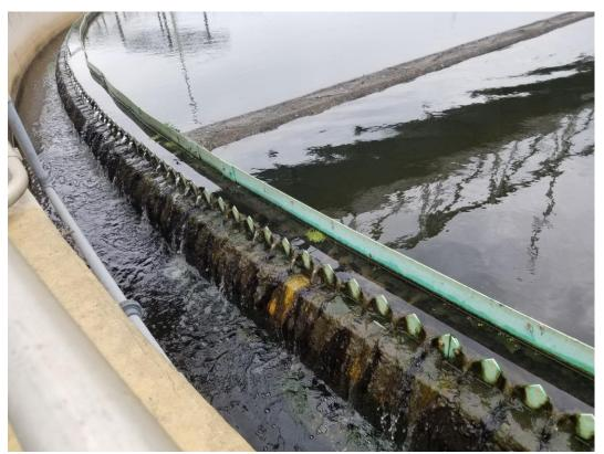
Picture 10: 6/14/23 – Secondary clarifier 7A was observed to have algae/vegetation growth along/past the weir.
