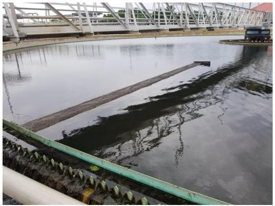
Picture 9: 6/14/23 – The scum trough at secondary clarifier 7A was observed to be clogged with scum.
