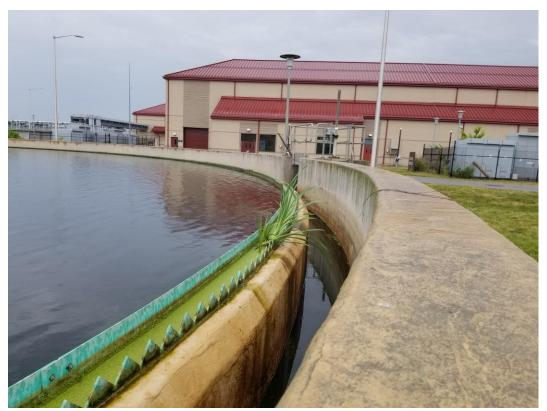
Picture 18: 6/14/23 – Secondary clarifier 6A was observed to have grass/vegetation growth along the weir.
