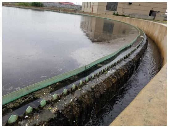
Picture 16: 6/14/23 – Secondary clarifier 5B was observed to have algae/vegetation growth along/past the weir.
