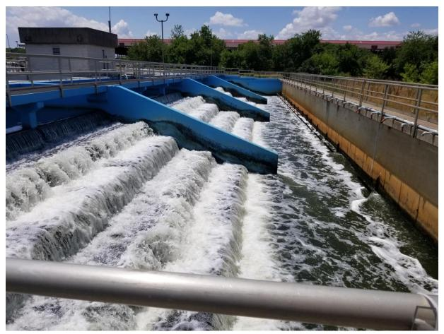
Picture 26: 6/14/23 – Final Effluent at the step aeration system.
