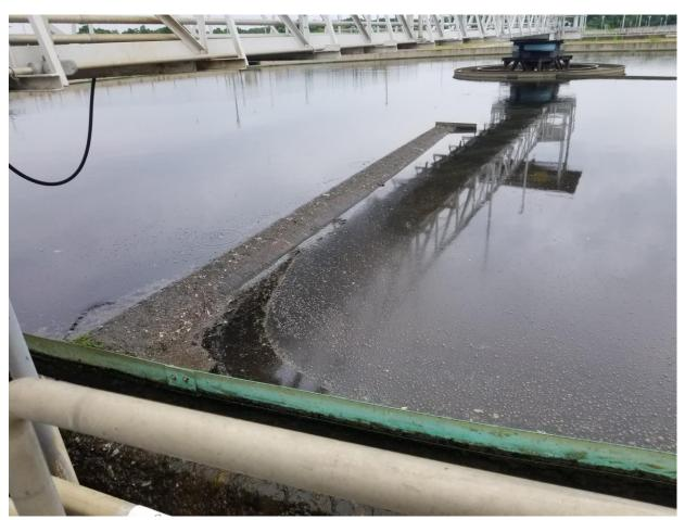
Picture 6: 6/14/23 – The scum trough at secondary clarifier 5A was observed to be clogged with scum.
