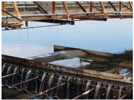
Picture 20: 6/14/23 – The scum trough at secondary clarifier 13B was observed to be clogged with scum.
