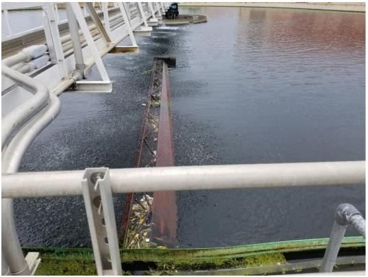
Picture 17: 6/14/23 – The scum trough at secondary clarifier 6A was observed to be clogged with scum.
