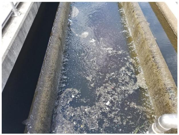
Picture 25: 6/14/23 - Solids and trash observed to be floating on water surface in the DNFs.
