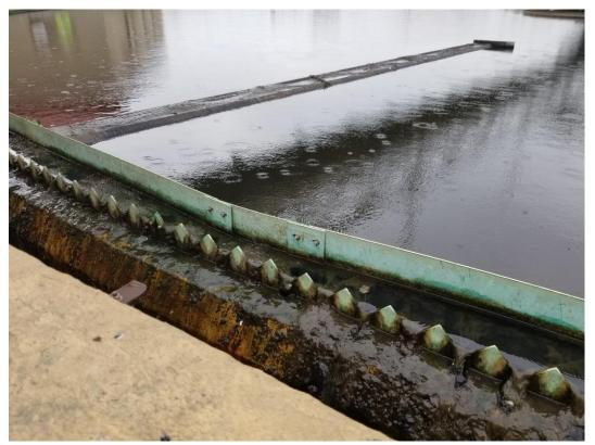
Picture 12: 6/14/23 – The scum trough at secondary clarifier 7B was observed to be clogged with scum.
