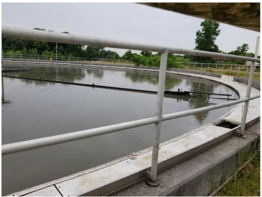
Picture 2: 6/14/23 – The PST #11 skimming arm was observed to be functioning, but should be adjusted as needed to function as designed.
