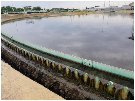
Picture 13: 6/14/23 - Secondary clarifier 7B was observed to have algae/vegetation growth along/past the weir.
