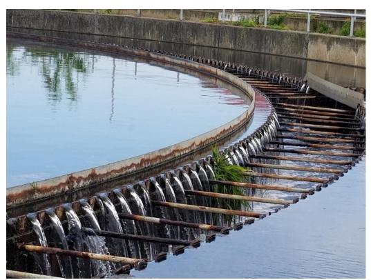
Picture 22: 6/14/23 – Secondary clarifier 13B was observed to have grass/vegetation growth along the weir.
