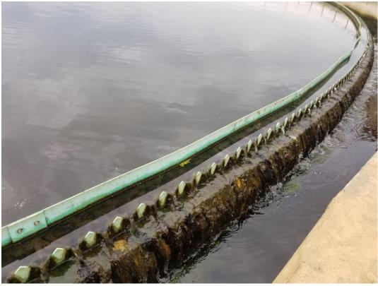
Picture 11: 6/14/23 – Secondary clarifier 7A was observed to have algae/vegetation growth along/past the weir.
