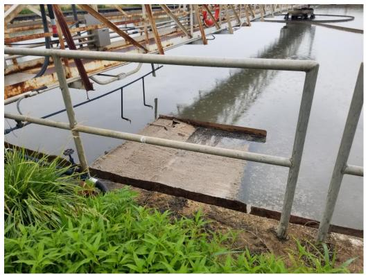
Picture 3: 6/14/23 – The scum trough at PST #1 was observed to be clogged with scum.
