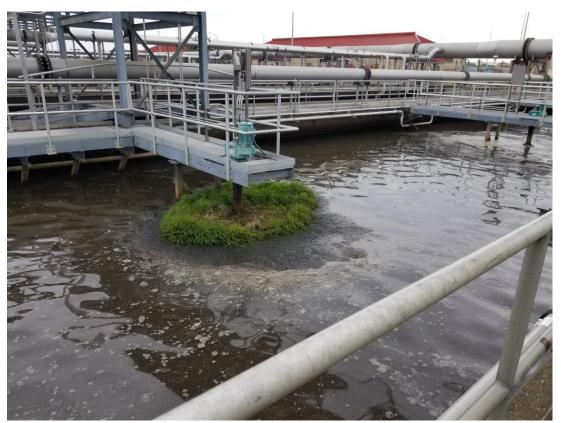
Picture 5: 6/14/23 – At ASP #2, vegetation was observed around one of the mixers at the reactor labeled 8A PASS.
