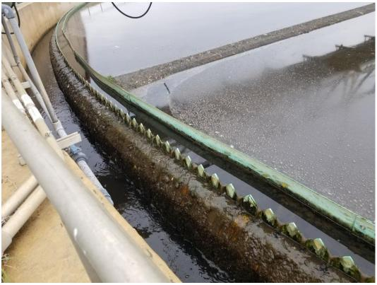
Picture 7: 6/14/23 – Secondary clarifier 5A was observed to have algae/vegetation growth along/past the weir.
