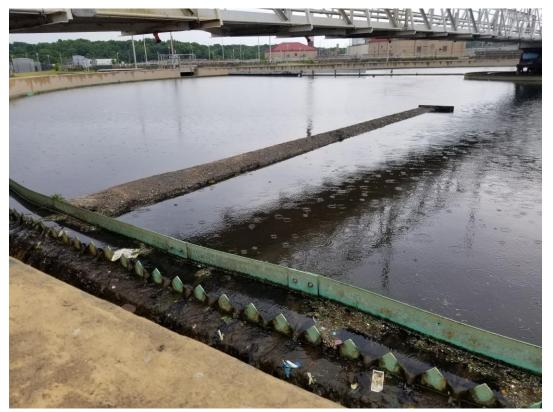
Picture 14: 6/14/23 – The scum trough at secondary clarifier 5B was observed to be clogged with scum.
