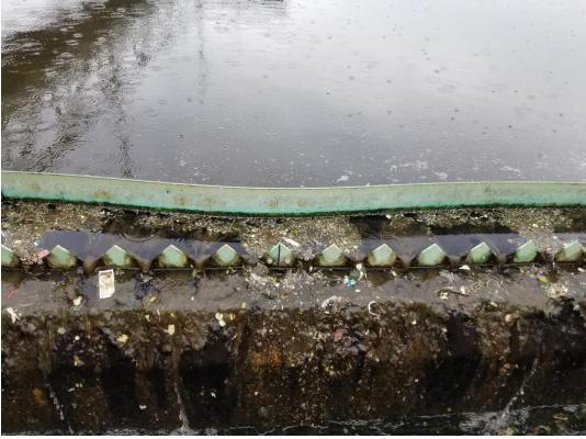
Picture 15: 6/14/23 – Secondary clarifier 5B was observed to have solids/trash debris leaving past the weir.
