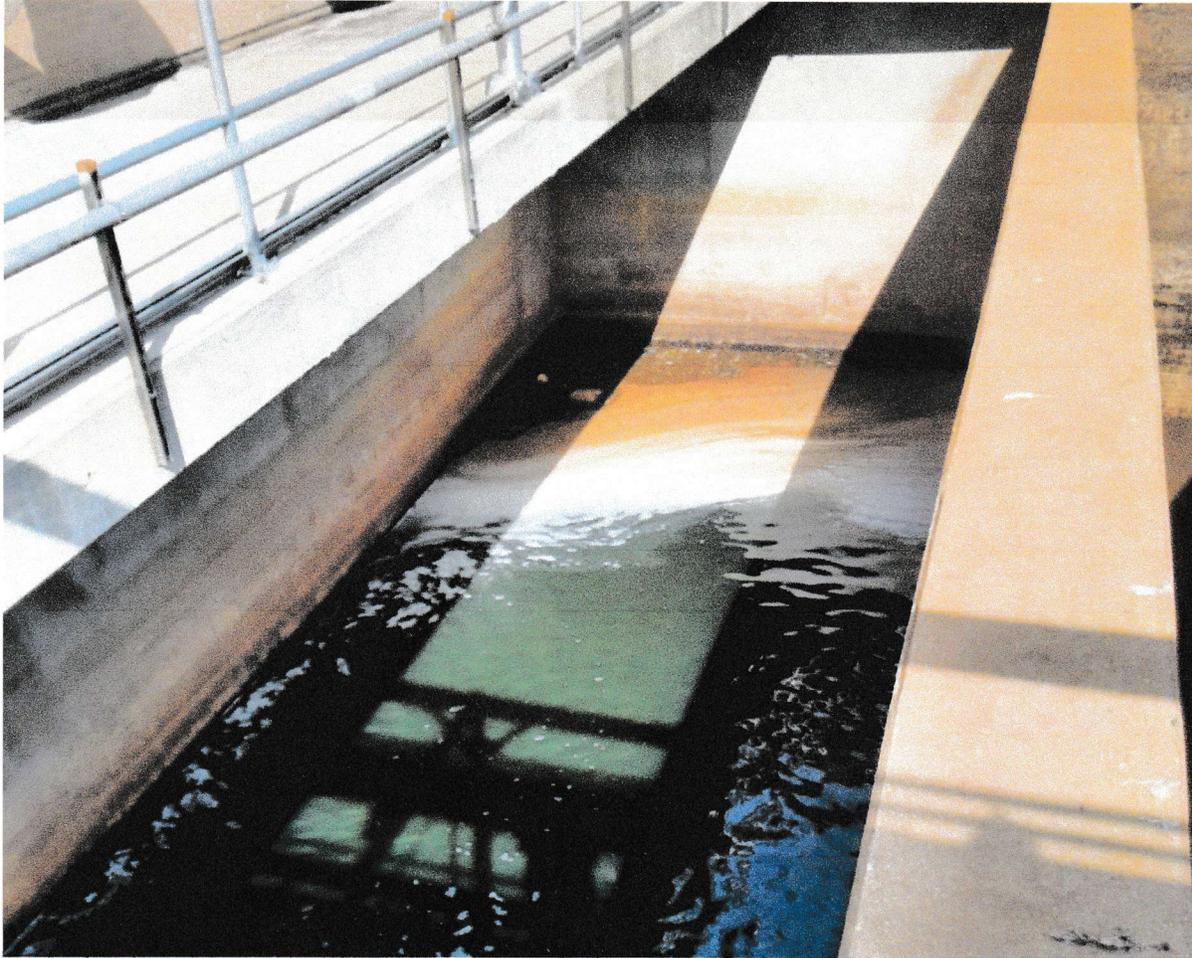
Picture #6 - 4/16/22 effluent from DNF at Clear well. Note floating remnants of scum, FOG and solids
