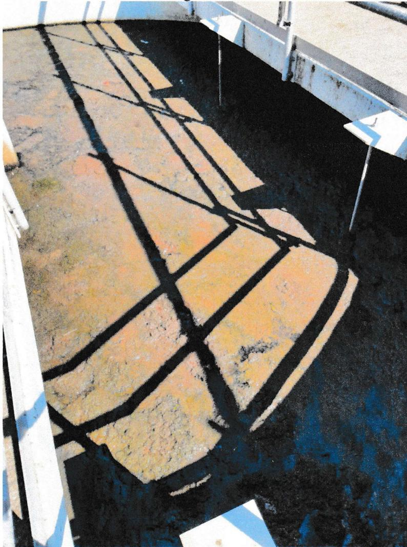
Picture # 2 - 4/16/22 Treated water from the sand filters that flows to the chlorine contact chambers
