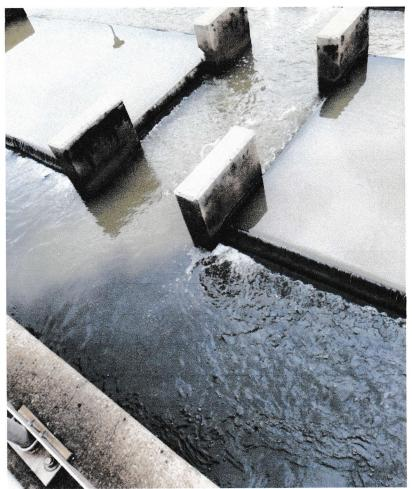
4/6/22 Dark grey effluent on the right is effluent from GSTs mixing with PST effluent. Color caused by 4,000 mg/L or higher TSS. This water is going to the biological reactors for secondary treatment.
