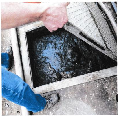
4/6/22 Sludge pit at GST was completely filled. The pit collects the sludge from the GST.
