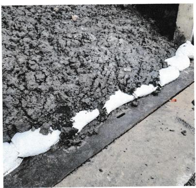
4/6/22 Sewage sludge overflowing the berm.
