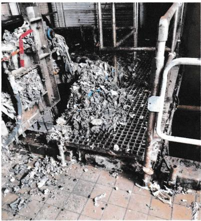
4/6/22 Trash overflowing the belt transport system
