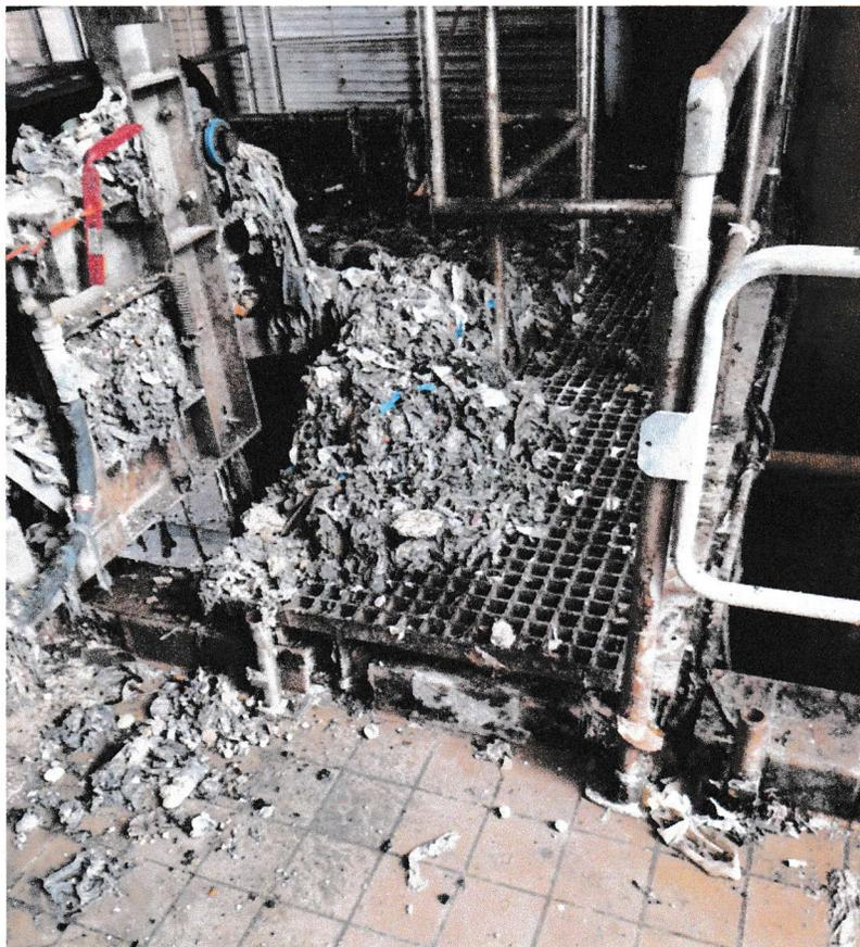
4/6/22 Trash overflowing the belt transport system
