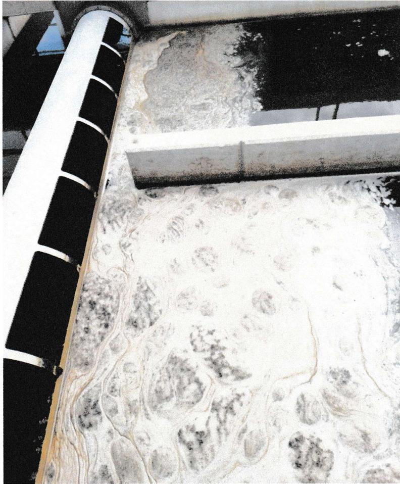
4/6/22 Heavy layer of scum at the chlorine contact chamber
