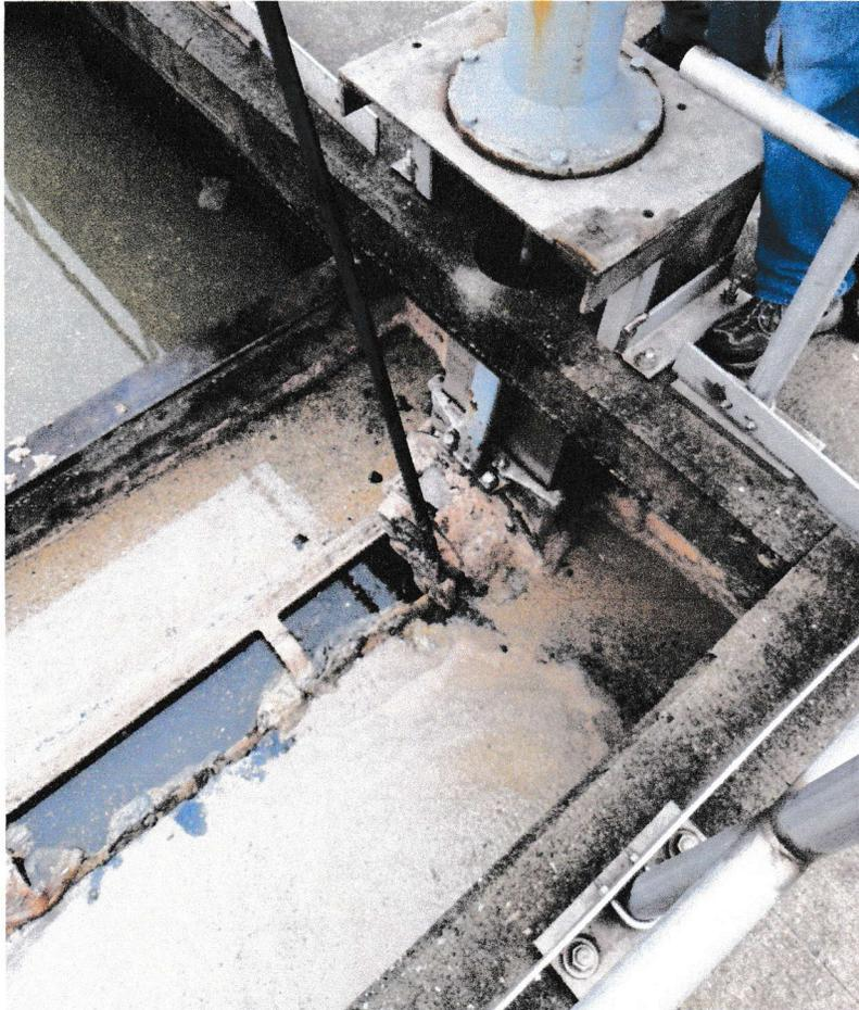
4/6/2022 PST scum trough requires turning. Mr. Thomas, from Hazen and Sawyer turns the scum trough with tool designed to rotate the trough.
