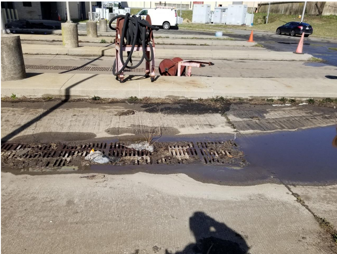
Picture 12: Trench drains were observed behind the dried sludge loading building.
