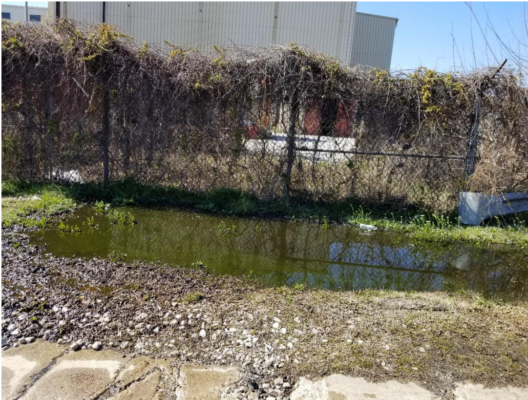
Picture 5: An oily sheen and green-ish color were observed in the flow water along the flow path from the pelletech building towards the dried sludge loading building.
