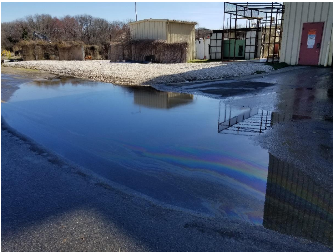
Picture 2: An oily sheen and green-ish color were observed in the flow water along the flow path from the pelletech building towards the dried sludge loading building.
