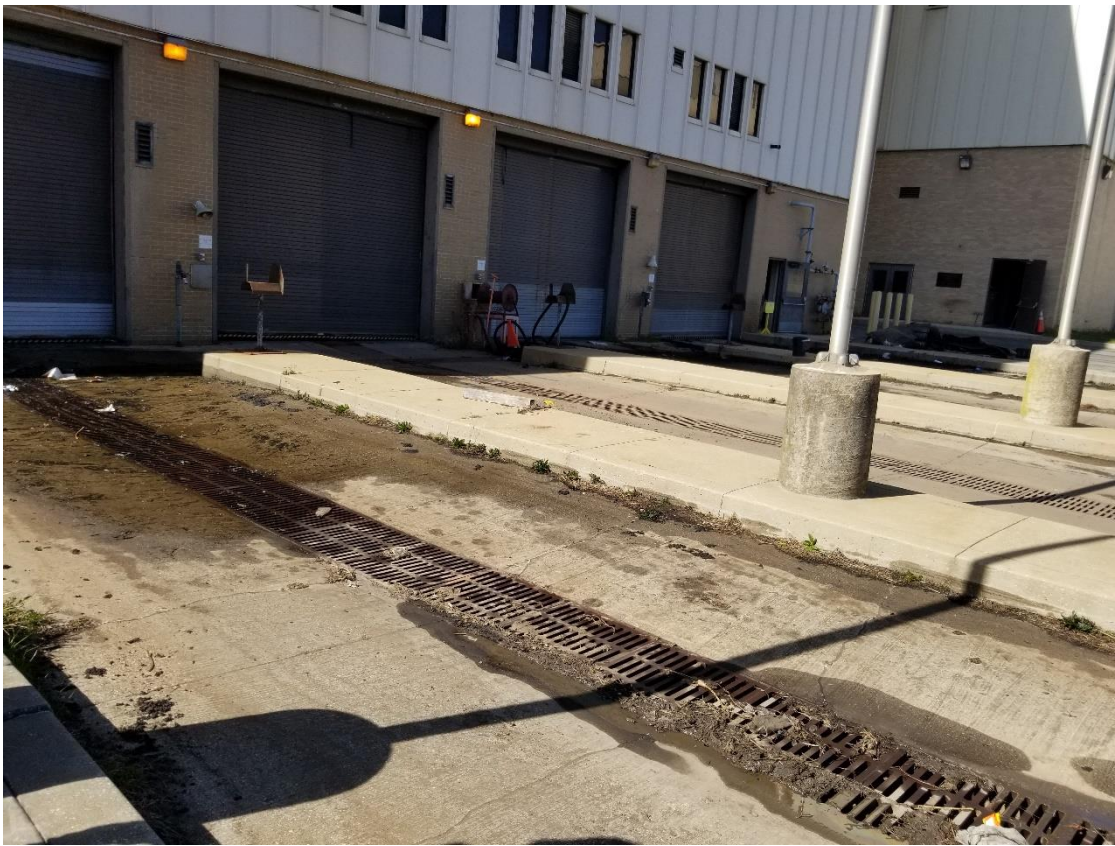
Picture 13: Trench drains were observed behind the dried sludge loading building.
