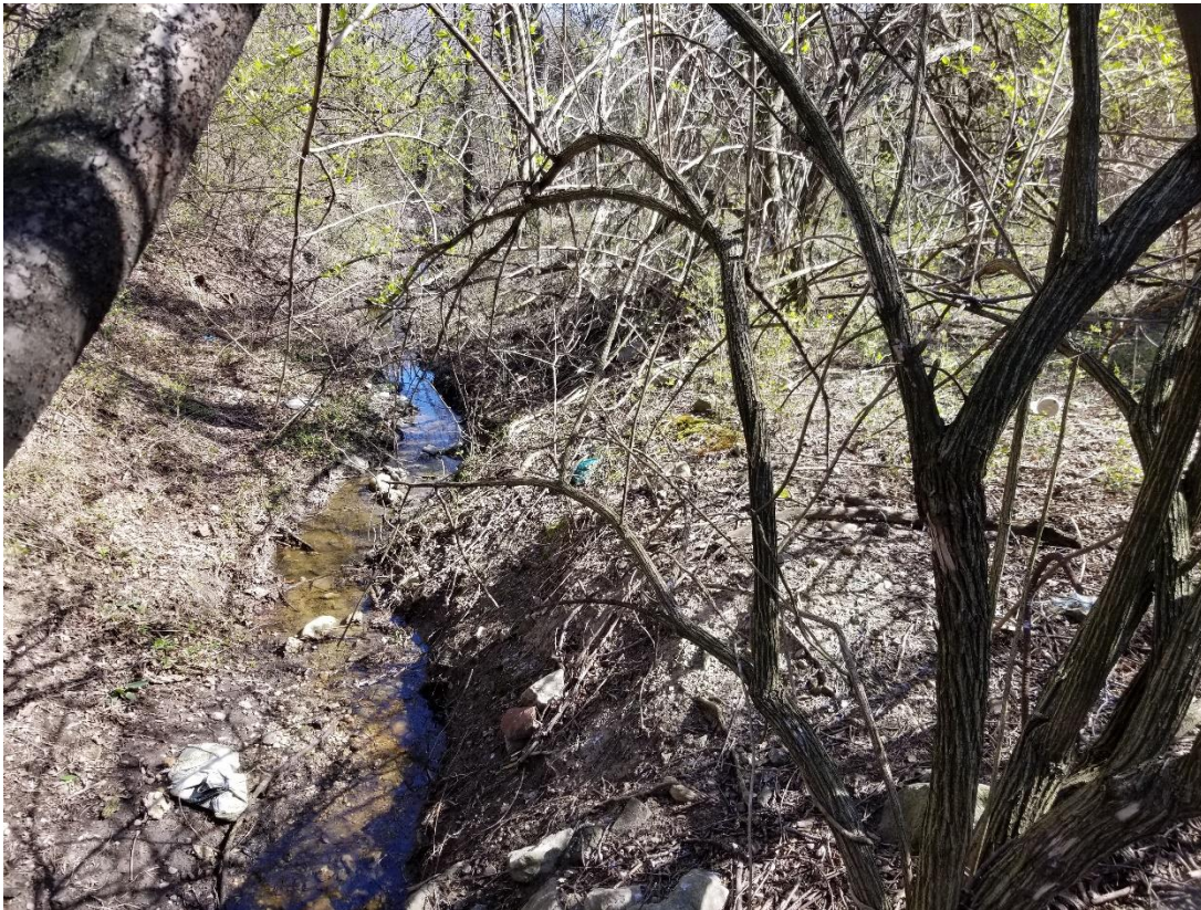
Picture 10: The flow (from the stormwater management culvert located south-east of the dried sludge loading building) leaving the site was observed to have an oily sheen.
