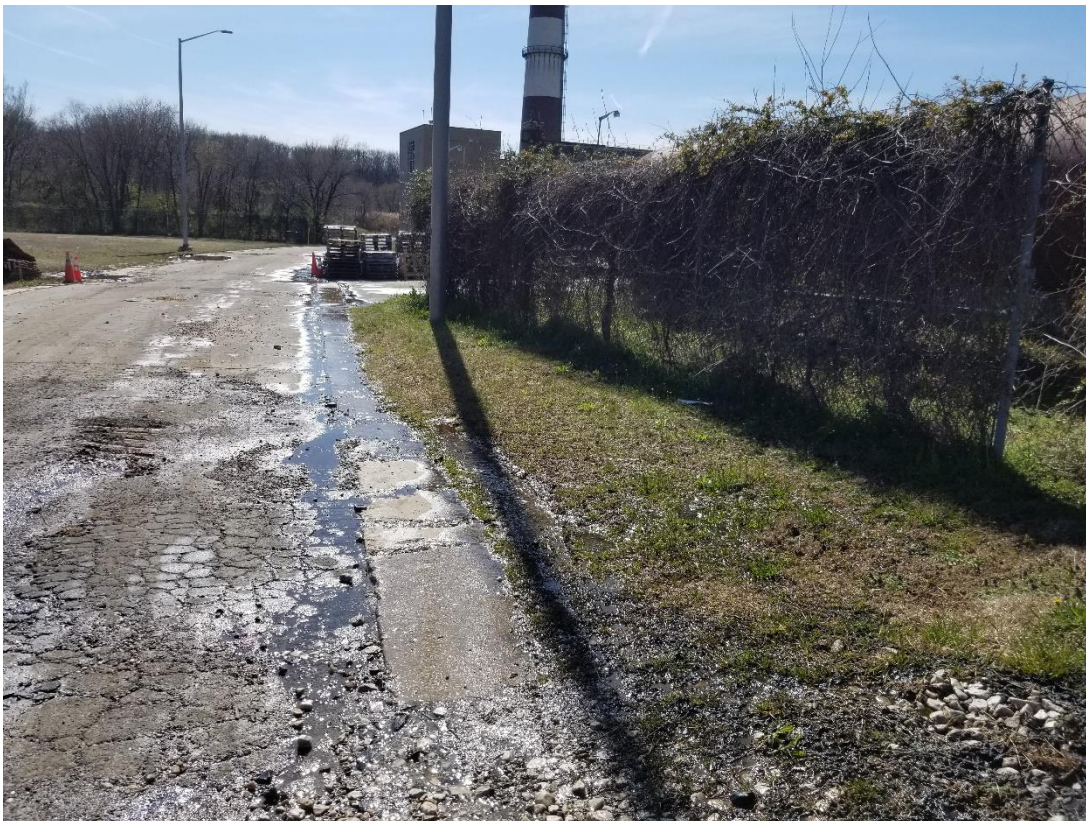
Picture 6: An oily sheen and green-ish color were observed in the flow water along the flow path from the pelletech building towards the dried sludge loading building.
