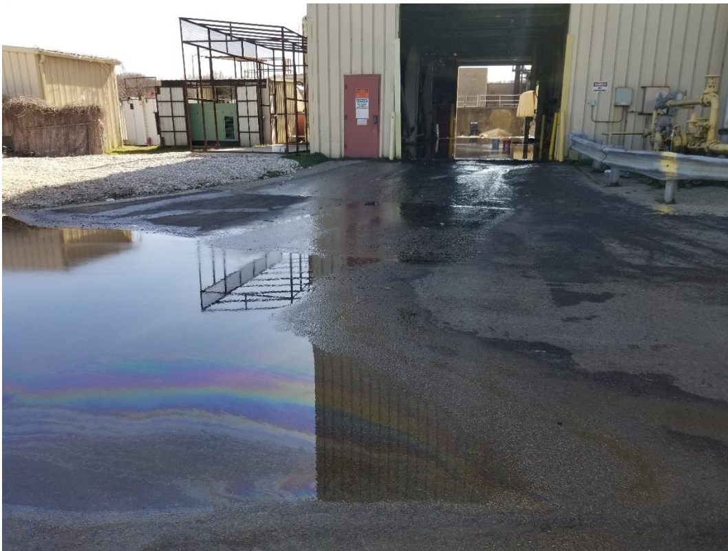
Picture 1: Water was observed flowing from the pelletech building. An oily sheen and green-ish color were observed in the flow water along the flow path from the pelletech building towards the dried sludge loading building.
