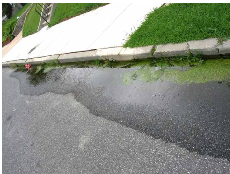
Dry weather discharge and algae in NSA-L-85
