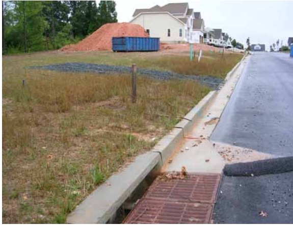
poor sediment control in NSA-L-177
