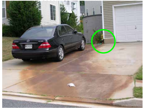
Impervious downspout drainage & staining in NSA-L-197
