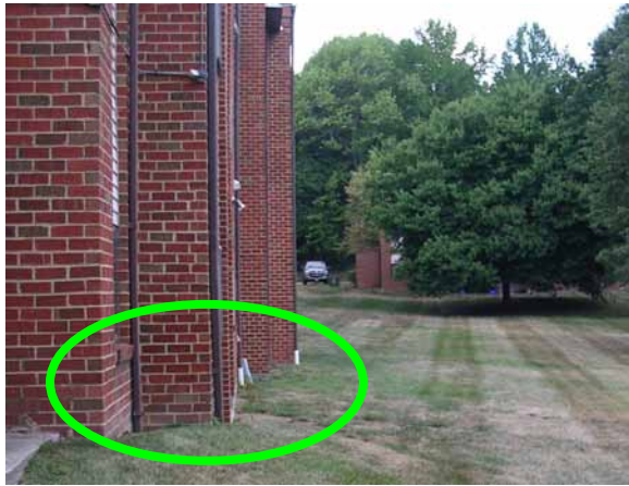
Directly connected downspouts in NSA L-155B that are suitable for redirection onto lawn
