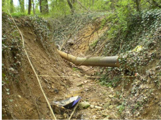
Figures 14A & B: Eroded areas in upstream reach of HW-08-00-01
