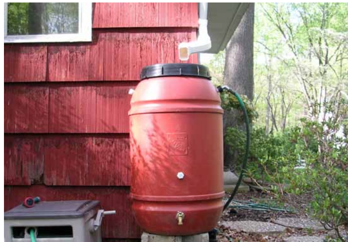
A typical rain barrel installation with overflow hose
