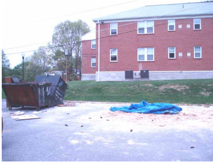
poor sediment control in NSA-L-89
