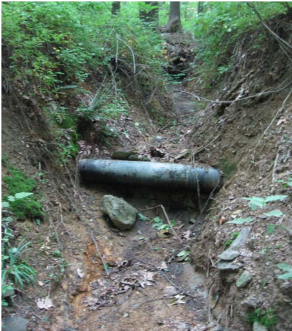
Figures 18A & B: Exposed utility and erosion in SR-08-02-01
