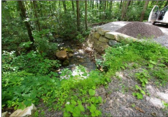
Figure 2. Passive treatment/limestone sand dump area.
