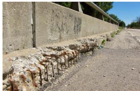
Figure 10. Example of car (top) and metal reinforced concrete (bottom) corrosion. Top image by ICPRB. Bottom image from McHenry County courtesy of Scott Kuykendall.
