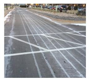
Figure 51. Example of anti-icing applied to roadways. Notice the ideal application is with bare pavement between lines. Image by MPCA from Flickr Commons.
