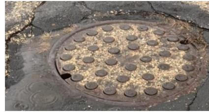
Figure 14. Example of corroded manhole cover and stormwater infrastructure frequently exposed to salt-rich stormwater. Image from [3].
