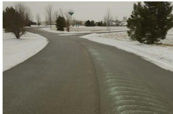
*Figure 73. Correct and overapplication of salt on the same road. Image from McHenry County Sensible Salting PPT.*
