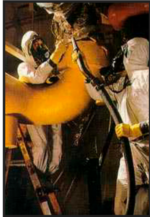
Asbestos Removal
