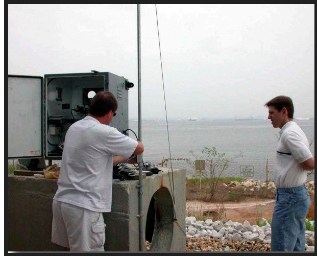
MDE Staff Installing Regional Haze Camera
