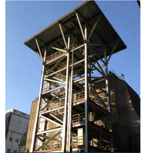
Hepo Facility, Shanxi
