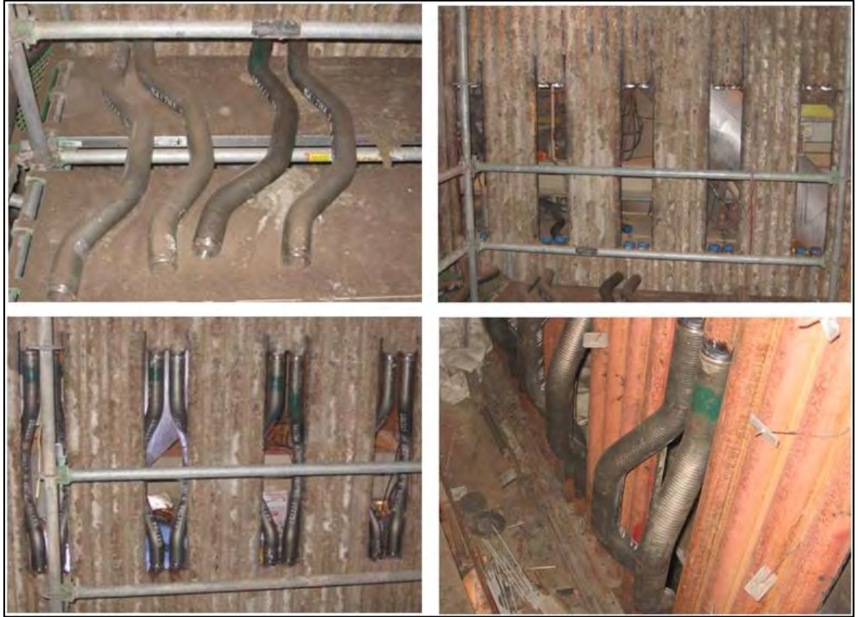
Figure 4. Waterwall Tube Modifications for Tertiary Air Nozzles
