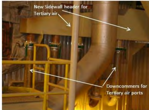
Figure 2. Tertiary Air Side Wall Header
