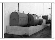
Figure 15 - Secondary Containment of Storage Drums behind a Car Repair Shop
