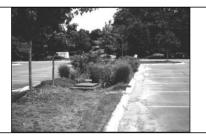
Figure 10 - Parking Lot Island Turned into Bioretention
