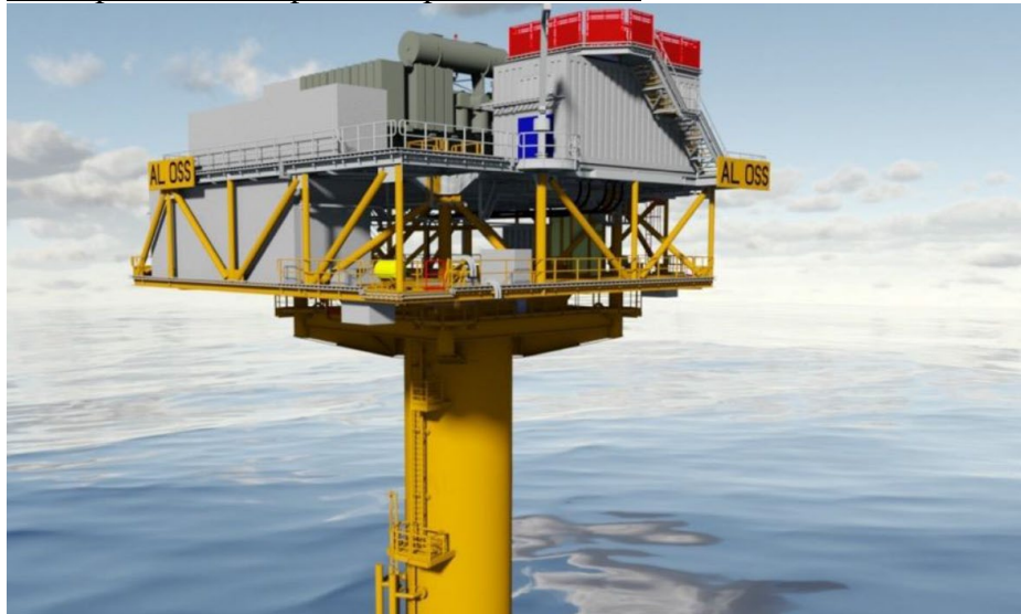
Conceptual OSS atop a monopile foundation
