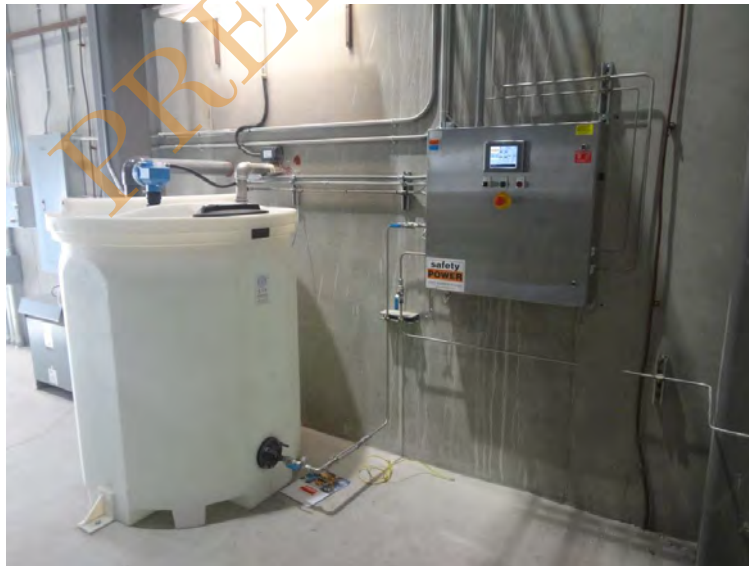
Figure 1 - Recommended tank/dosing panel arrangement
